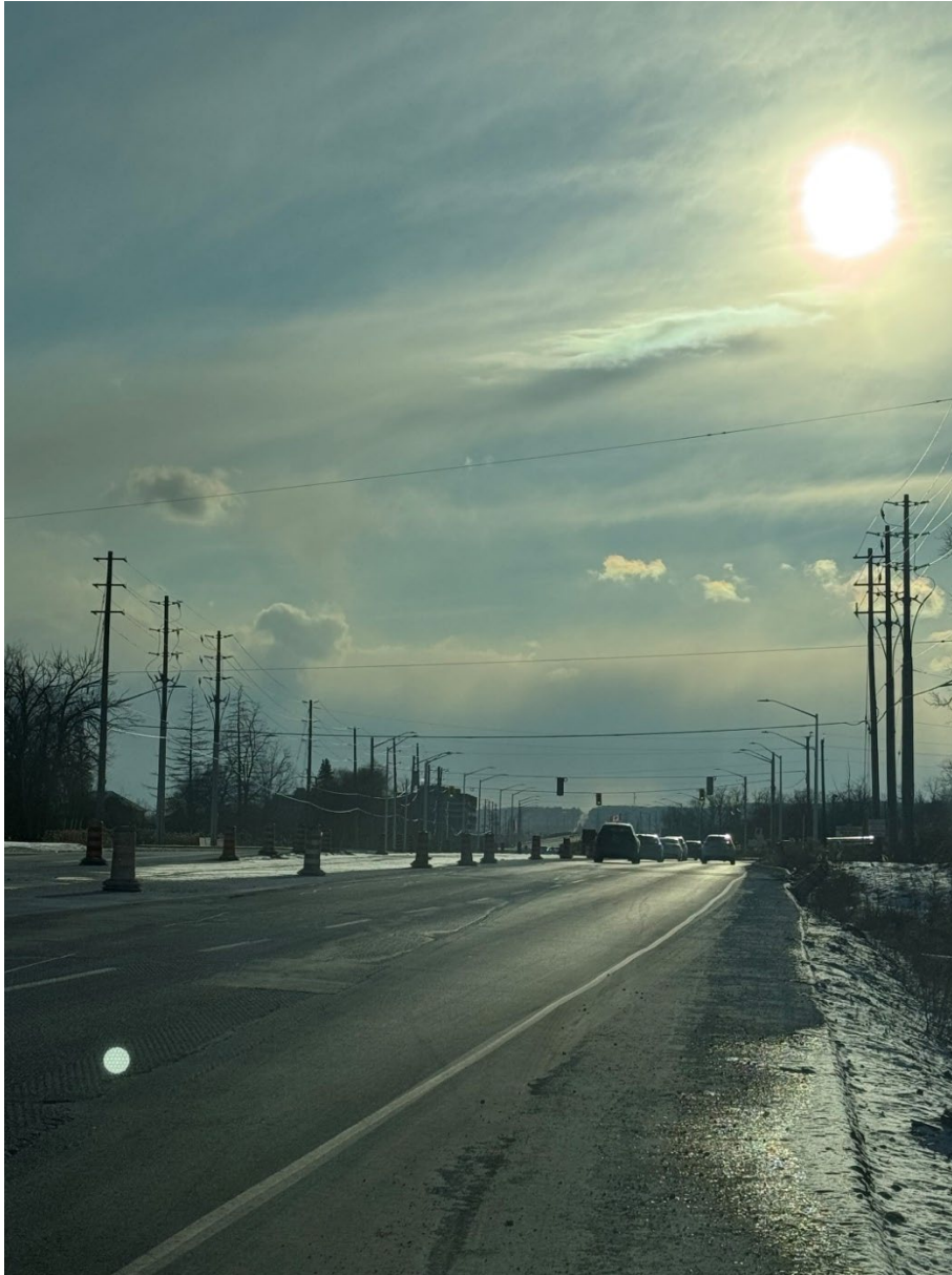
Figure 3 – 2021 Dundas Street Road Widening Project
