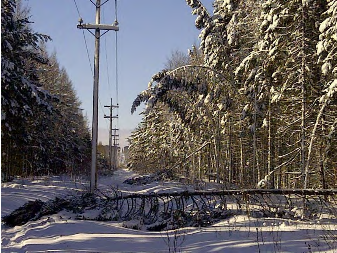
Figure 1: Express Feeder ROW - Trees under snow load
