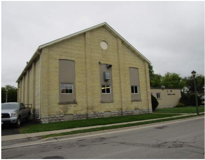
General view, west elevation of the 1920's Building
