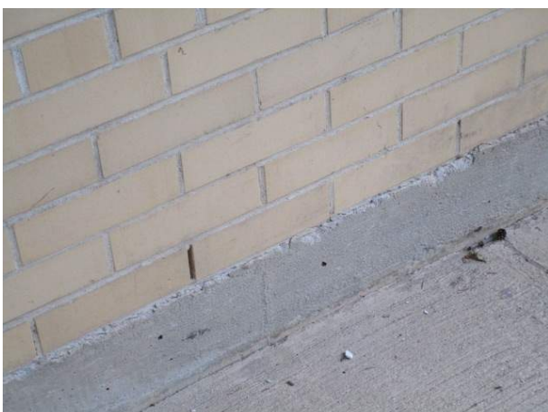
Weeping hole – brick masonry wall
