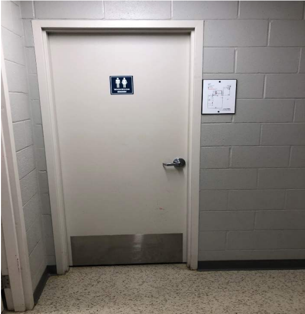
Painted Block Wall Covering / Painted metal door frame
