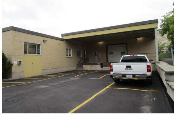
Loading dock area adjacent to single storey office building.
