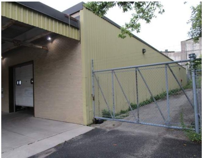
South elevation – 1950's Building Prefinished metal siding
