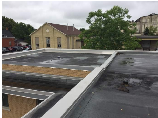
1992 Addition / 2006 Upper roof area.
