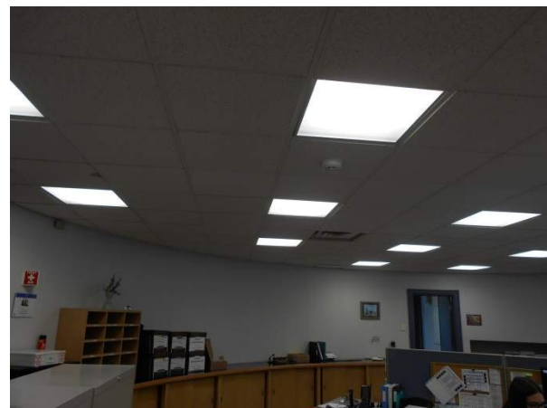
2'x2' Recessed Light Fixture
