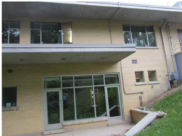
Large overhang, lower level and upper level.
