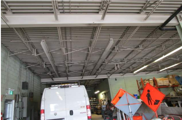
Roof structure of east truck bay
