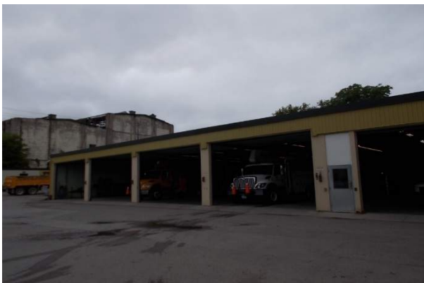
East truck bay and warehouse building
