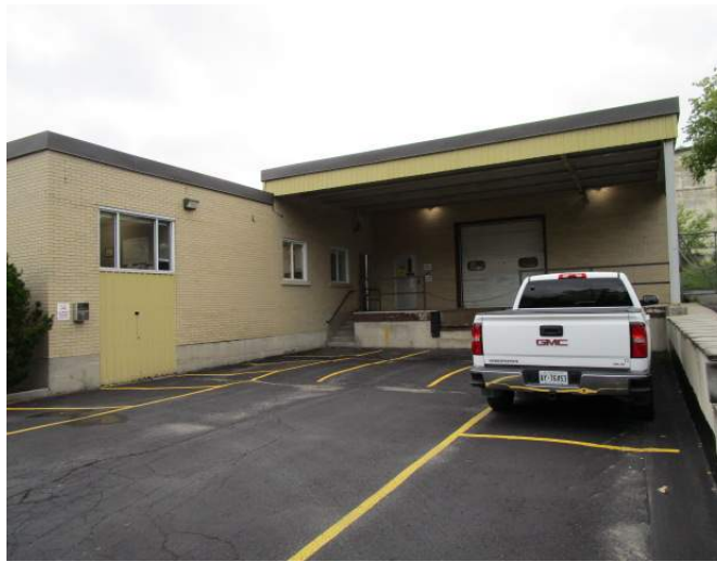
Loading dock – 1950's Building
