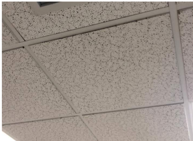
Ceiling Finishes – Acoustic Tile
