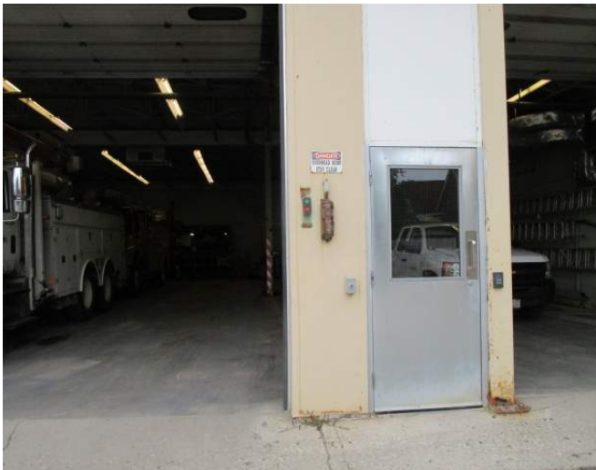
Metal door to garage area of the 1950 Building
