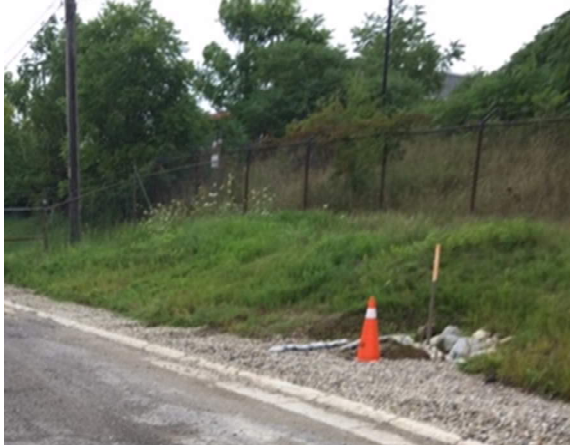
Chain link fencing
