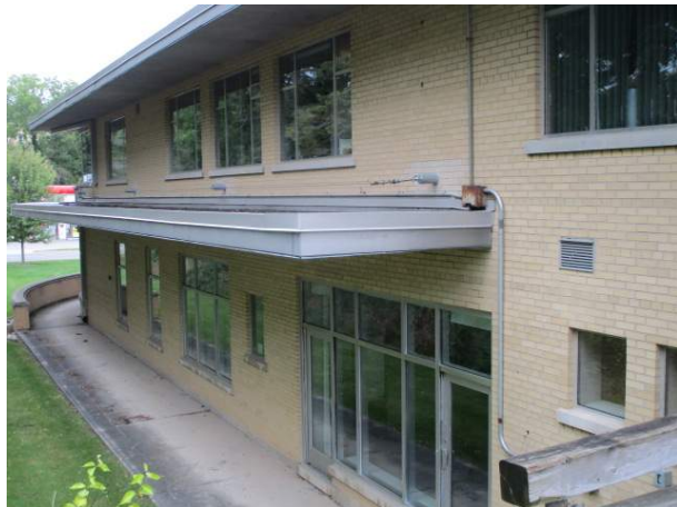
Windows/board room doors, south elevation
