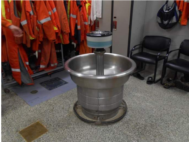
Round sink in office area washroom
