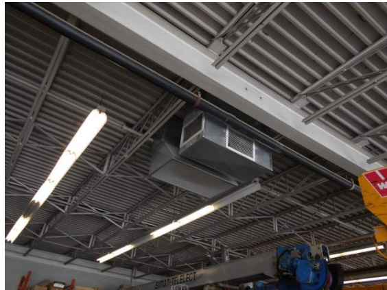
Ceiling Hung Light Fixtures
