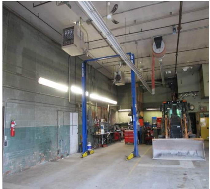
Flooring - Exposed Concrete
