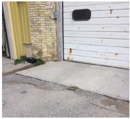
Concrete apron at entrance to garage area.
