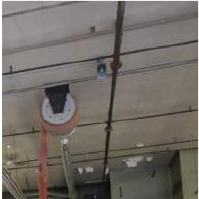
Ceiling - Ceiling Board (1920's section of building)
