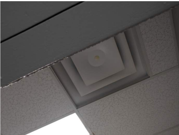
Rectangle ceiling diffuser
