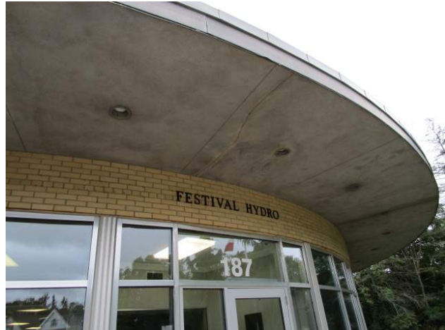
Exterior Recessed Light Fixture
