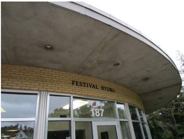
Large overhang – soffit constructed with transite panels
