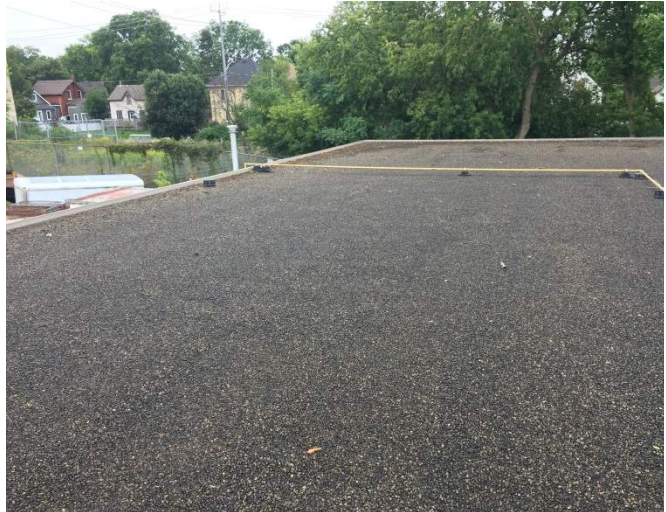
Built up asphalt roof over vehicle garage area, 1950's Building
