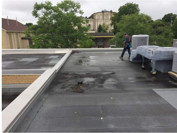
Upper roof area – repairs completed in 2014(?).
