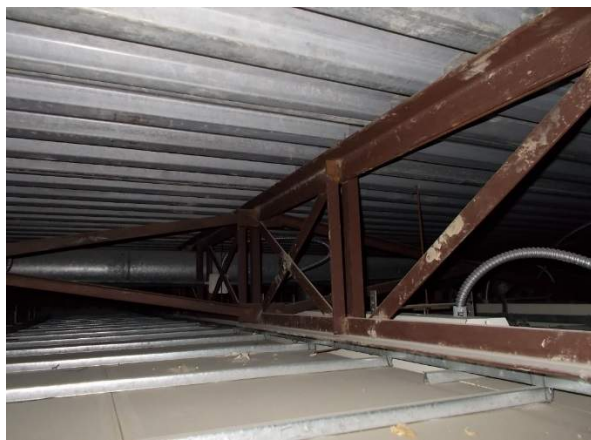
Roof raming of original section
