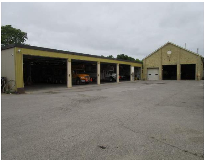
North elevation / 5 overhead doors & 1 man door – 1950's Building
