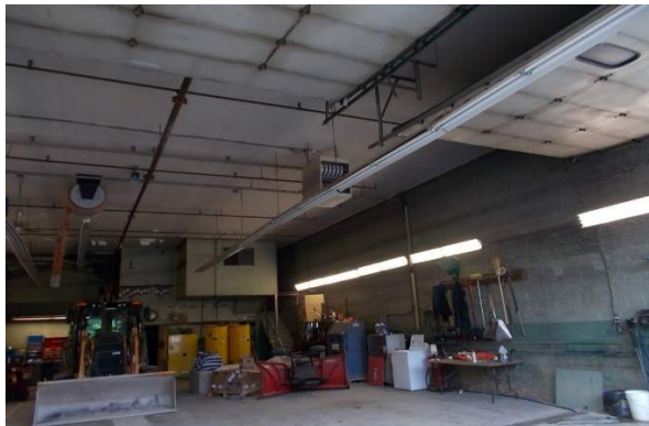
Interior of north truck bay building.
