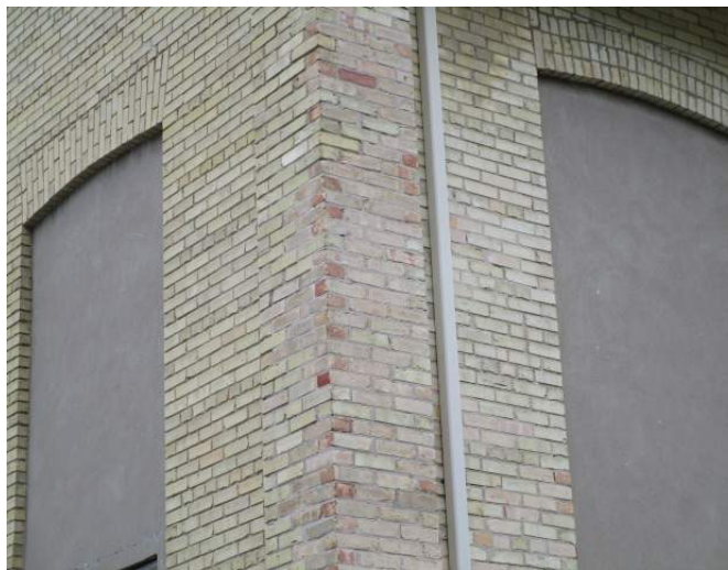
Previous brick masonry repairs – 1920 Building
