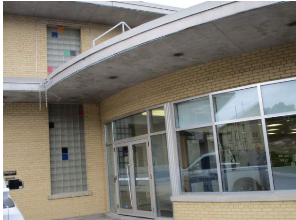
Double door, staff entrance / glass block feature wall.
