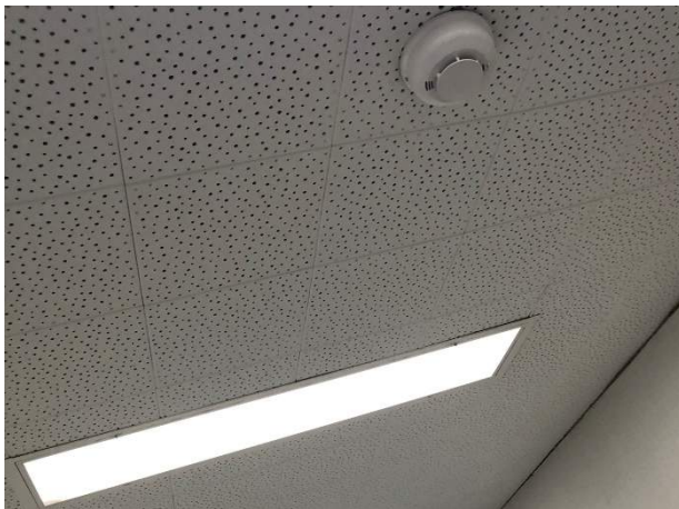
Ceiling Finishes – Acoustic Panel
