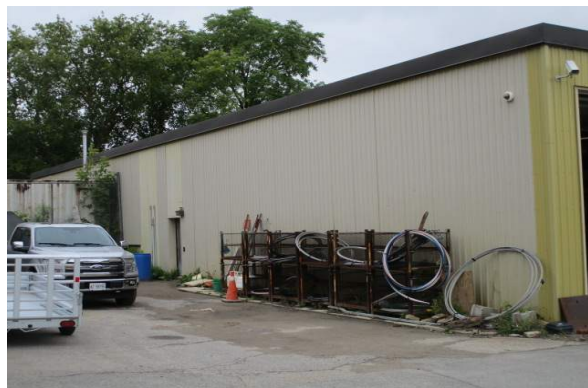
Siding covering the north truck bay and warehouse building.
