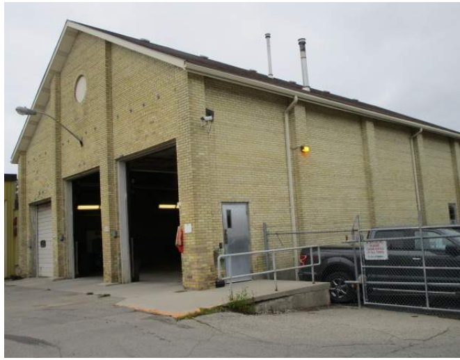
North and east elevation – 1920's Building
