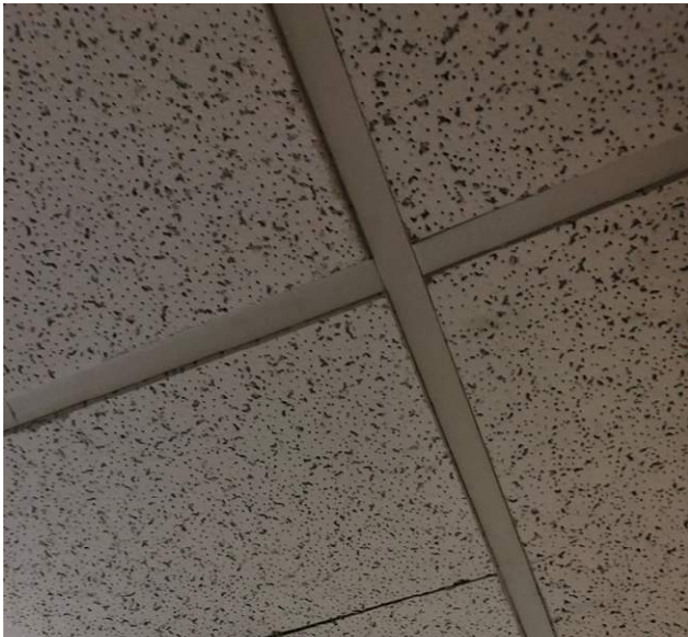
Ceiling – Suspended Ceiling Tile
