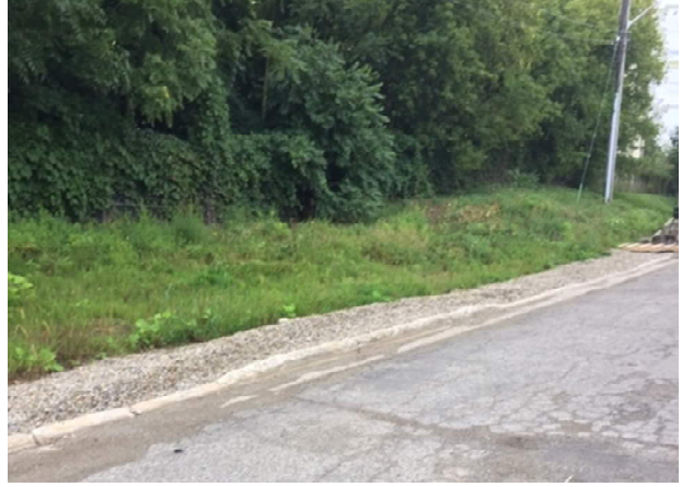
Overgrown chain link fencing
