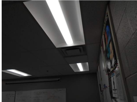
2'x4' Recessed LED Light Fixture
