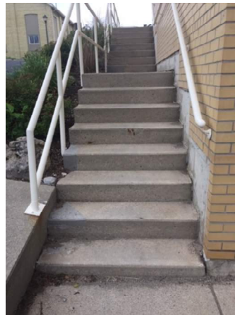
North-east stairwell to ground level at Wellington St.
