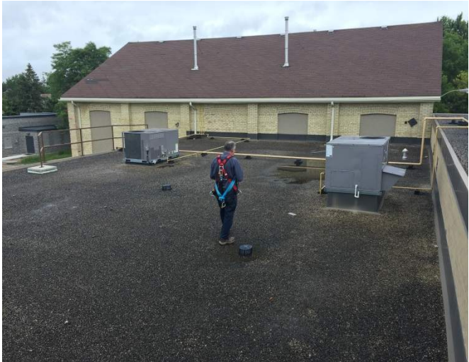
Shingled roof on 1920 Building, built – up asphalt roof over office area, 1950 Building.
