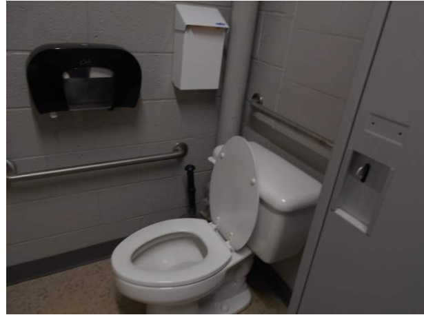
Barrier free washroom in office area
