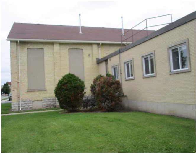
South elevation, 1920's building / west elevation, 1950's Building
