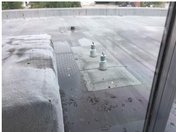
Low roof area – roof anchors added
