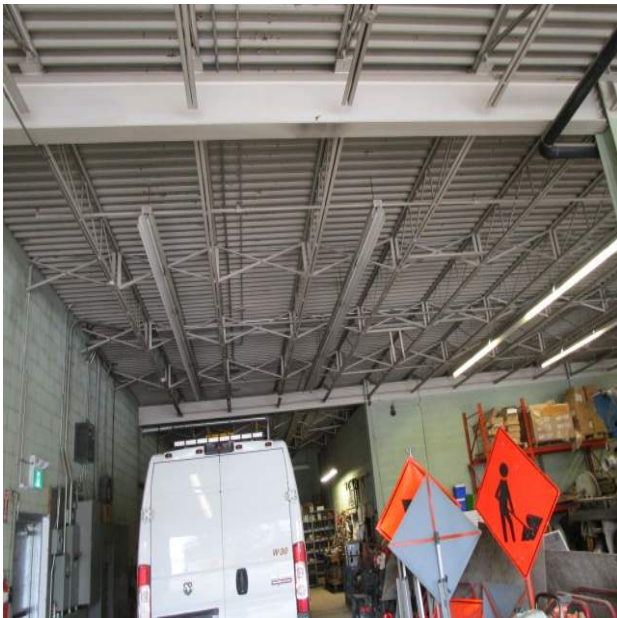
Ceiling – Exposed Painted Metal Deck
