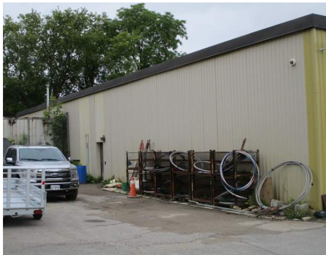
East elevation – 1950's Building Pre-finished metal siding.
