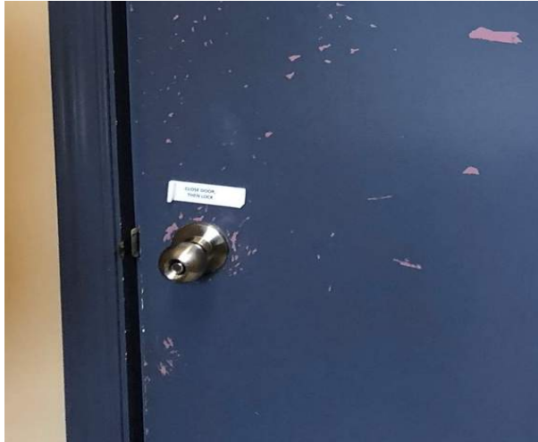
Interior Doors – Painted Finishes
