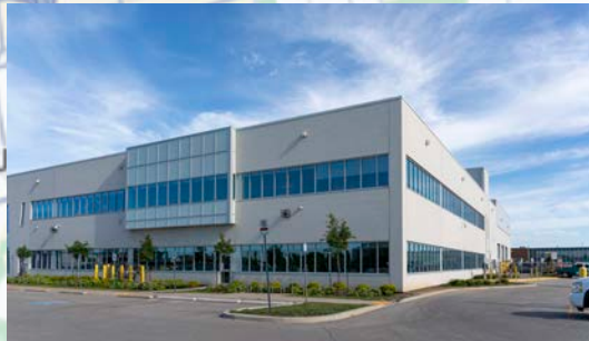
Toronto Hydro 71 Rexdale Blvd. 2016
