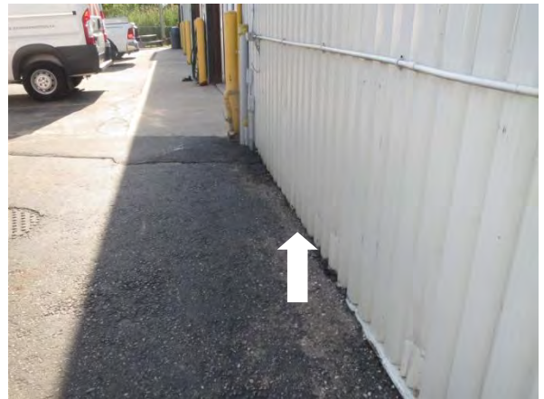
Repair: Asphalt over Metal Siding Location: outside Meter Shop
