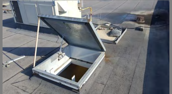
Roof Hatch Location: Over second Storey Office
