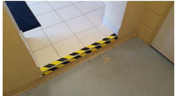
Sample: Floor level Transition Location: Stair No. 1
