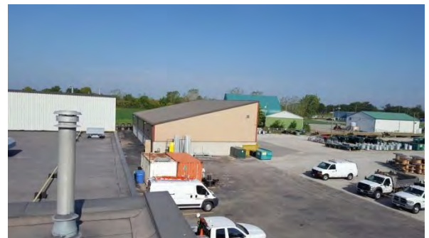
Pitched metal roof Location: Works Garage
