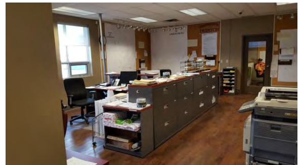
Sample: flooring in good condition Location: First Floor Open Office Area
