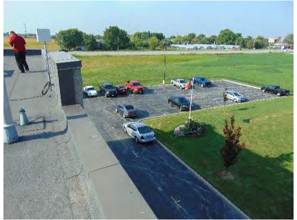
View of South-West Parking Lot
