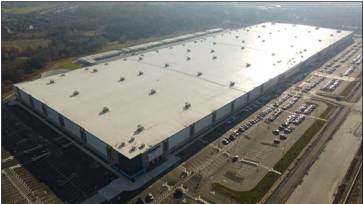
Recently Completed TPO Project
