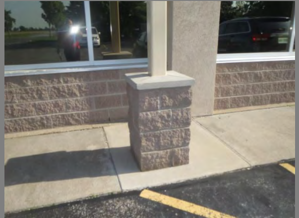
Sample: Masonry Pier | Sidewalk Location: South Wall
