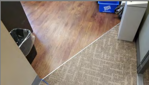
Sample: Floor transition in good condition Location: First Floor Open Office
