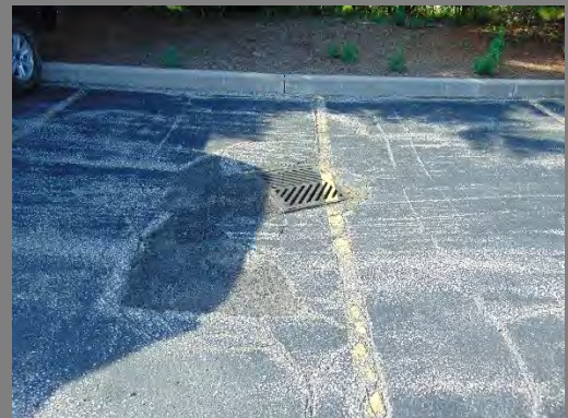
Catch Basin Location: South Parking Area
