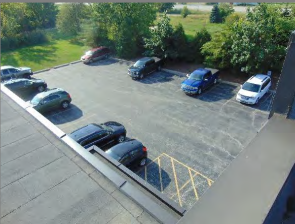
View of South-East Parking Lot
