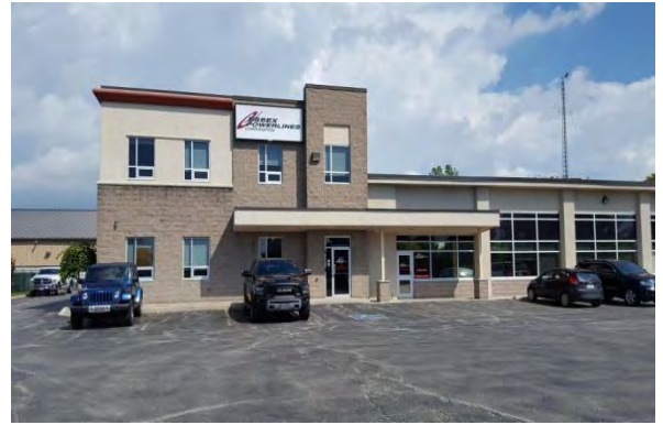
Sample: South Façade, EFIS and Masonry Location: South Facade
