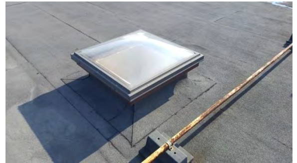
Skylight Location: Over Second Floor Office
