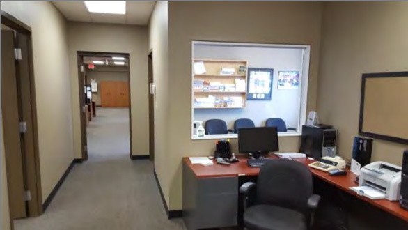
Sample: Flooring, Walls, in good condition Location: Reception
