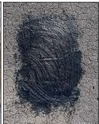
Core Cut Patched
