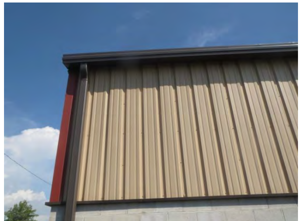
Sample: Siding in good Condition Location: Works Garage
