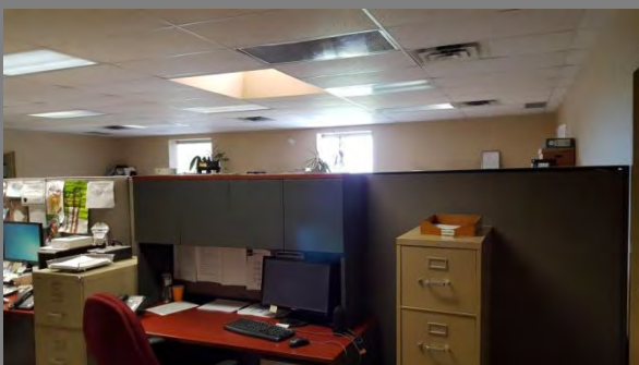
Sample: Demountable partition in good condition. Location: Second Floor Office
