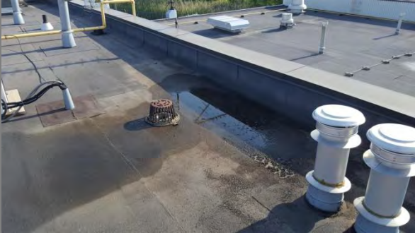
Roof Drain Clear – Small Ponding Location: Over Second Floor Office
