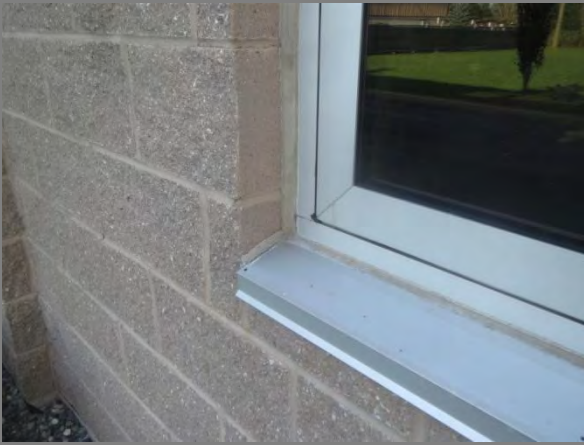
Sample: Window and Caulking in Good shape Location: Southwest Wall
