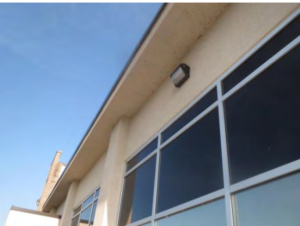
Sample: EFIS in good condition Location: South Wall
