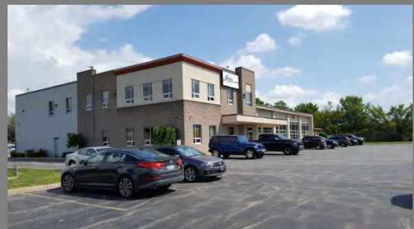
Sample: Metal Siding, EFIS and Masonry Facade Location: Looking at Main Entrance
