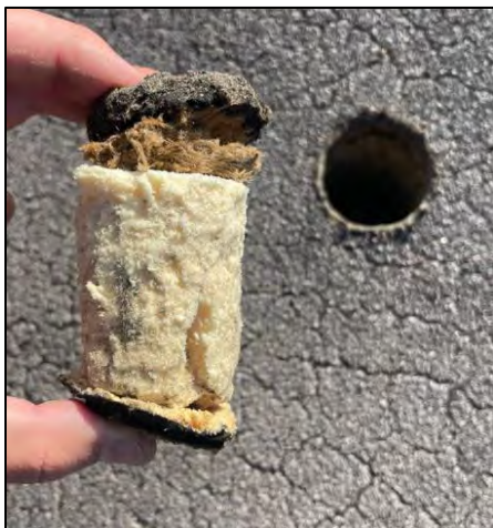
Core Cut of Roof System
