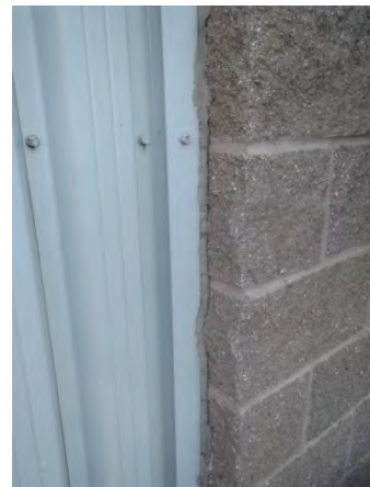
Sample: Caulking at Metal Siding | Masonry Location: West Wall
