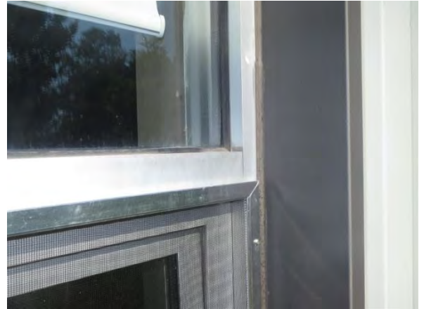
Sample: New window at Training Room Location: New Training Room
