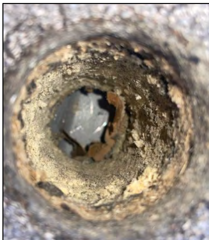
View of Metal Decking
