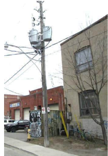
P27 – Guying Installation
