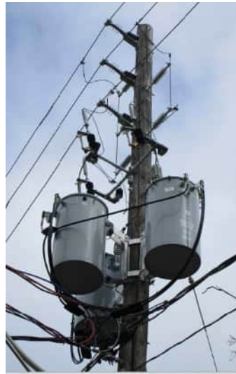
P27 OT24584 – 3-PH Transformer Installation
