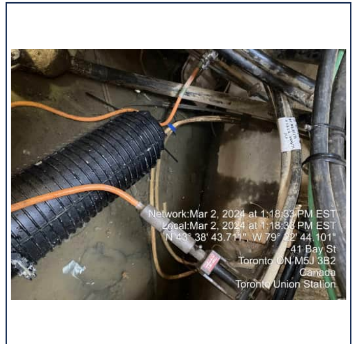
Spike Tool Installed
