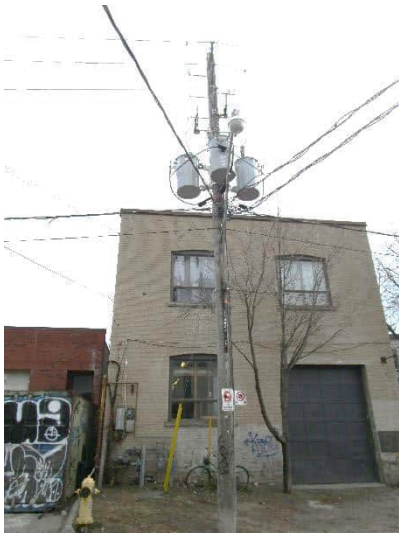
P27 OT24584 – 3-PH Transformer Installation
