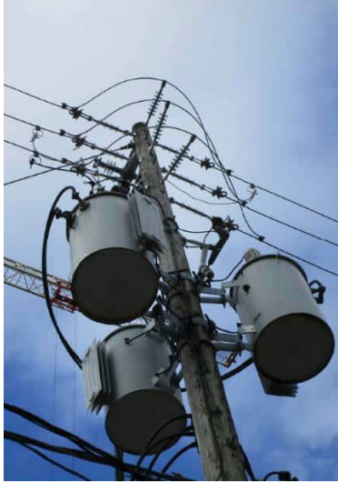
P58 OT400445 – Overhead Conductors Installation
