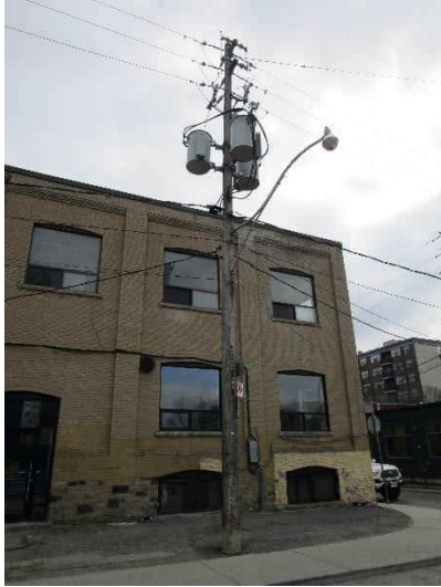
P58 OT400445 (Existing) – 3-PH Double Dead-End Configuration
