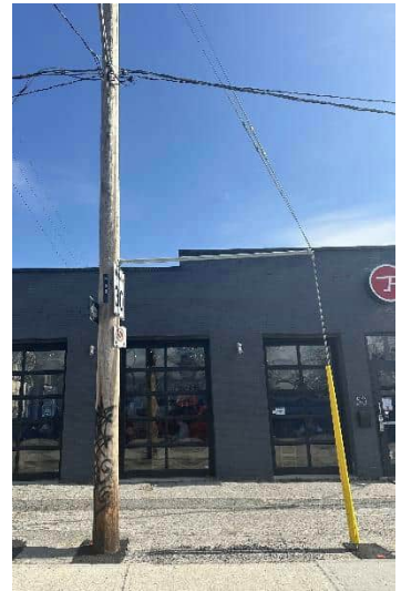
P50 – Pole Installation (Stenciling Issue Fixed)
