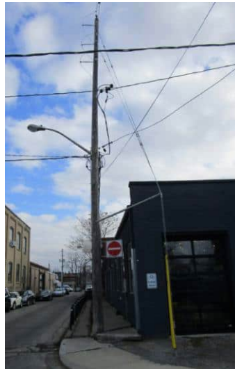
P11 (Existing Pole) – Guying Installation
