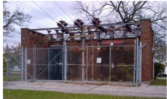
Figure 7: Residential Area MS (rear view)
