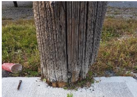
Figure 3: Rot at Base of a Pole
