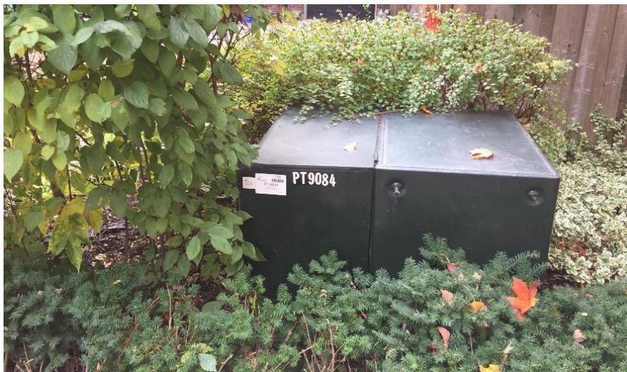
Figure 16: Padmounted Transformer Requiring Vegetation Removal
