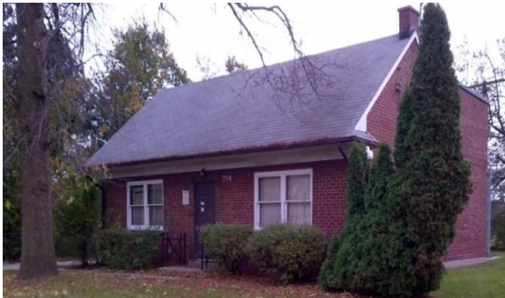
Figure 6: Residential Area MS (front view)
