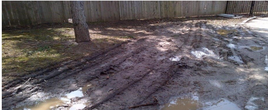
8 Figure 12: Damaged Landscaping
