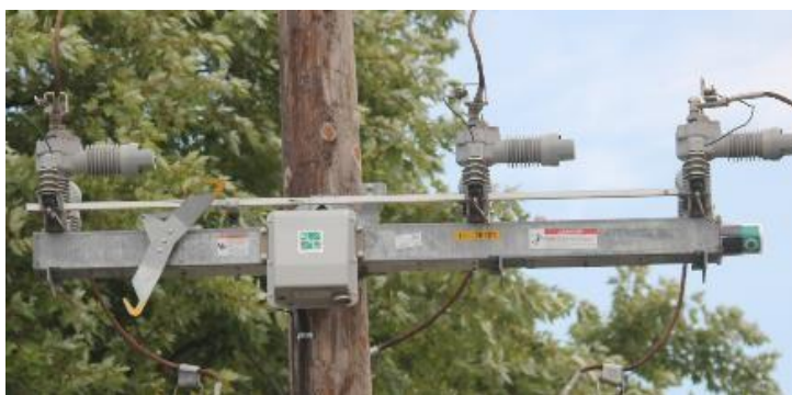
14 Figure 7: SCADA-Mate Switch
