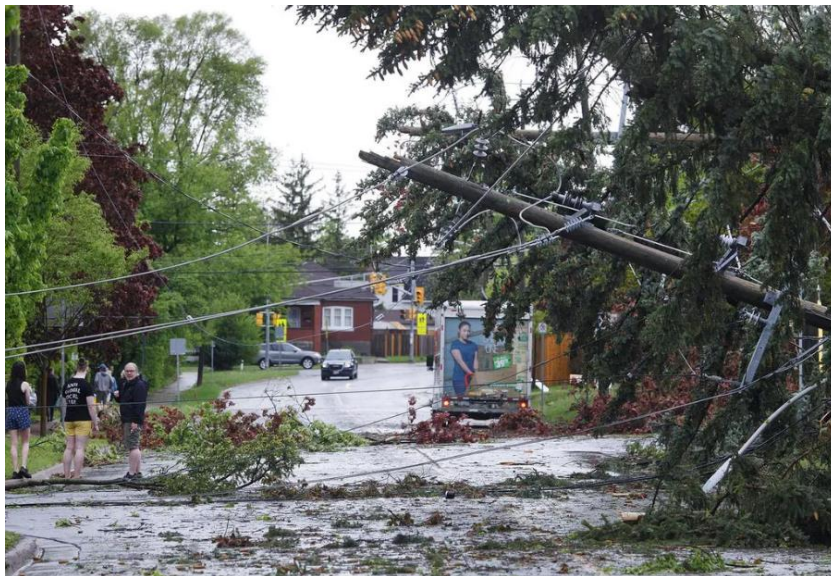
2 Figure 1: Damage caused by derecho wind storm in May 2022
