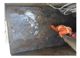
**Figure 10: Deteriorated Vault Floor**
