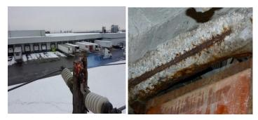
16 Figure 4: Pole fire caused by Tracking (left), Exposed and rusted rebar in Network Vault (right)
