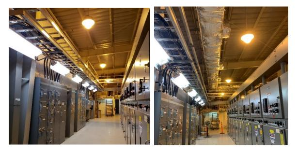
Figure 14: Examples of HVAC additions at Stations: Cavanagh Station without additional air conditioning (left) and after with ducts and venting installed for keeping air temperature and equipment cool (right).
