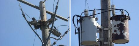
Figure 10: Animal Contact on Metal Switch Bracket (Left)/Rusted Overhead Transformers at Risk of
