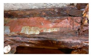
Figure 8: Corroded I-beams
