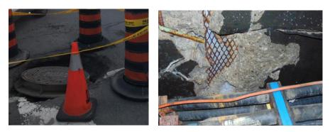
Figure 14: Cable Chamber Roof in HI5 Condition (Left), and Roof Inside View (Right)
