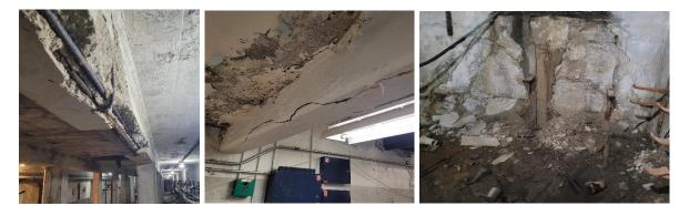
Figure 16: Examples of existing stations in critical condition, from left to right: George and Duke Station, beam with exposed rebar, Defoe Station cracked beam, Junction Station deteriorated foundation wall.
