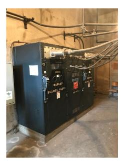
Figure 34: Example of Legacy Switchgear
