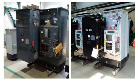
Figure 1: Snapshot of a Ventilated Network Unit (L) and Submersible Network Unit (R). The black protector is of a submersible design, which prevents water ingress.
