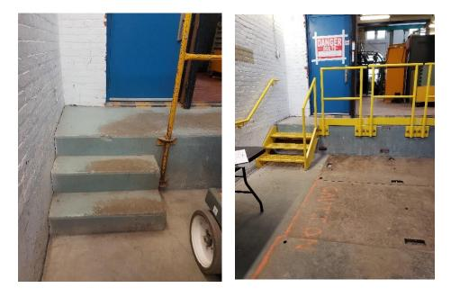
1Figure 9: Example of Terauley Station, replacing non-code-compliant stairs and railings with2functional ones, and improved dock access.
