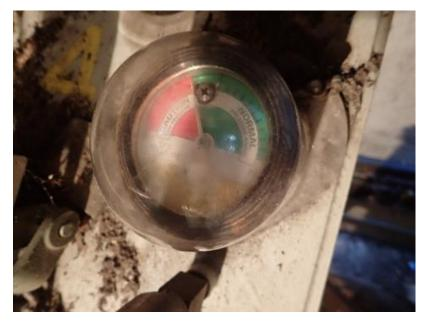
Figure 27: Example of a SF6 Switch with a "Low SF6" Reading
