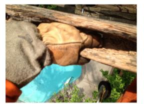
Figure 7b: Poor condition pole in close proximity to swimming pool
