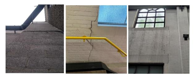
Figure 6: Examples of envelope deterioration at stations, from left to right: Glengrove Station
