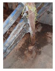
Figure 28: Example of Switch Supports that have rusted
