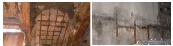
Figure 7: Roof and Wall with Exposed Rebar
