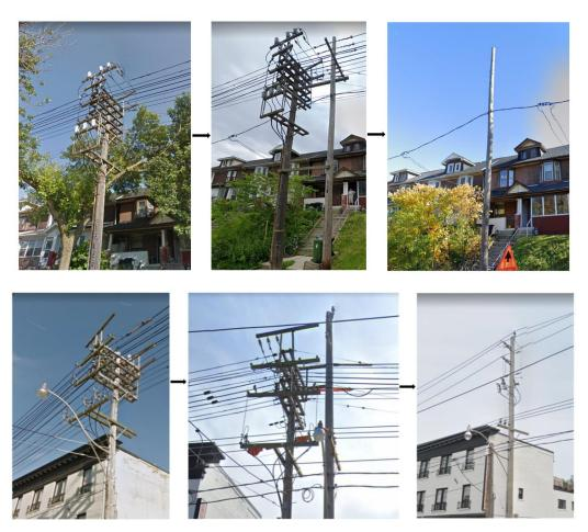
Figure 10: Actual box construction conversion project on Gerrard Street East at two locations. Photographs on the left show 4.16 kV box construction poles prior to conversion. Photographs in the middle are demonstrating the in-construction stage. The completed project is shown in the photographs on the right, where all 4.16 kV box construction has been removed.
