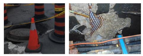
1 Figure 11: Cable Chamber roof in HI5 condition (left), Cable chamber roof inside view (right)
