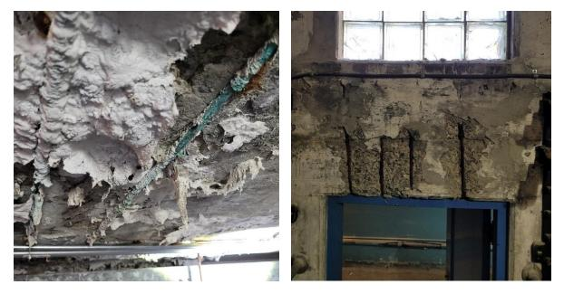
Figure 3: Examples of structural deterioration at stations, from left to right: Wiltshire Station exposed and corroded rebar with significant water infiltration, Wiltshire Station exposed rebar in concrete wall.
