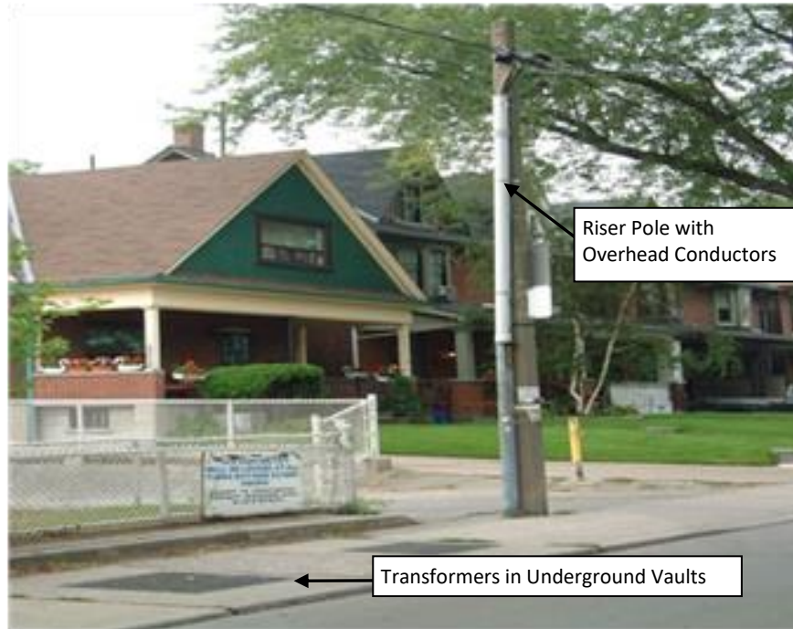
Figure 18: Typical Layout of Underground Residential Distribution
