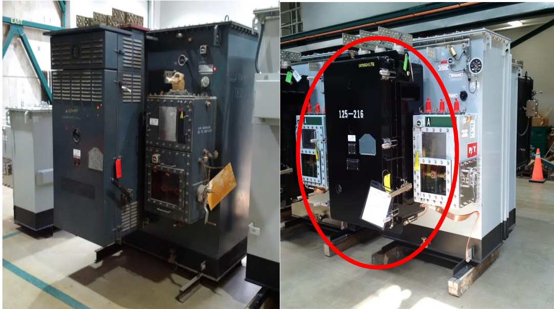
Figure 26: A ventilated Network Unit (Left) and a Submersible Network Unit (Right)
