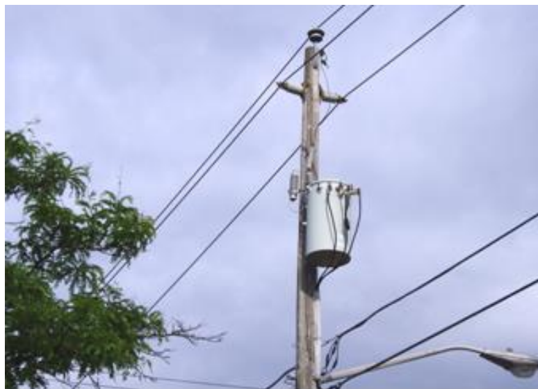
Figure 13: Overhead Distribution Transformer
