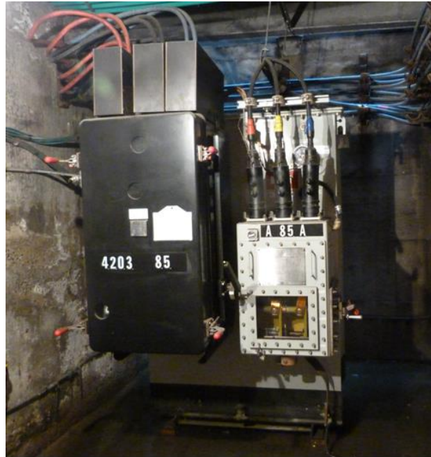
Figure 23: Submersible Network Unit
