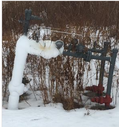
Figure 5.2-68: The Joule-Thomson Effect on a District Station
