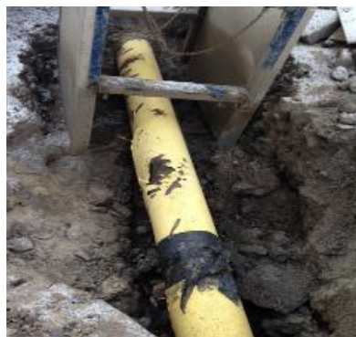
Figure 5.2-52: Multiple corrosion sites on NPS 12 St. Laurent pipe
