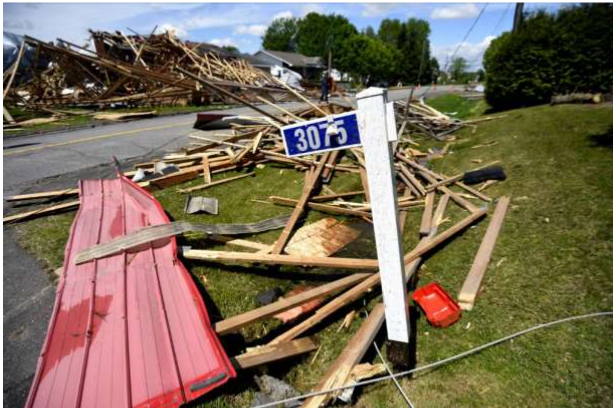
The remains of the roof of a hardware store that lifted off and crashed into neighbouring houses during a major storm is seen spread across residences in the community of Hammond in Clarence-Rockland, Ont., Monday, May 23, 2022. THE CANADIAN PRESS/Justin Tang Justin Tang.
