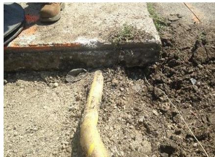
Figure 5.2-8: Shallow and embedded gas main due to road grade change
