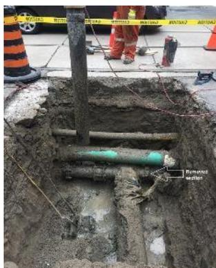
**Figure 5.2-22: Leak investigation on vintage NPS 12 gas main**
