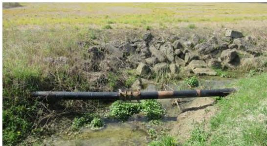
**Figure 5.2-13: Aerial crossing with exposed mechanical fitting**
