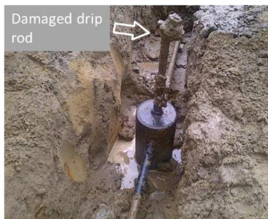
Figure 5.2-12: Damaged drip rod on vintage NPS 2 gas main
