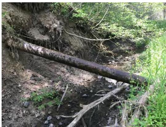
**Figure 5.2-15: Erosion increasing the unsupported length of an aerial crossing**
