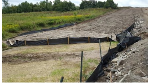
September 8 subsoil sediment deposition at toe slope from water erosion adjacent to creek
