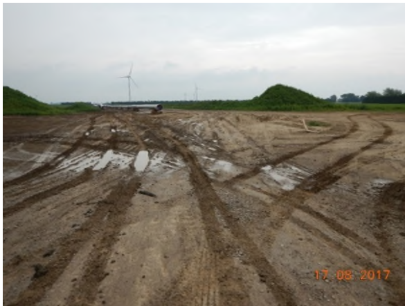
Aug 17 - P33 random pickup truck traffic in wet soil and through standing water
