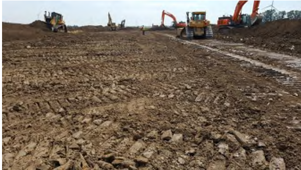
June 22 - P45 topsoil stripping with 12 heavy equipment machines and 3 tractor implements
