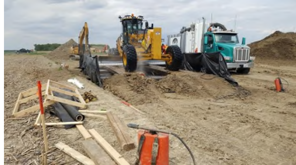
May 23 - P98 wash station cleaning infected SCN topsoil from machinery adjacent to non SCN field
