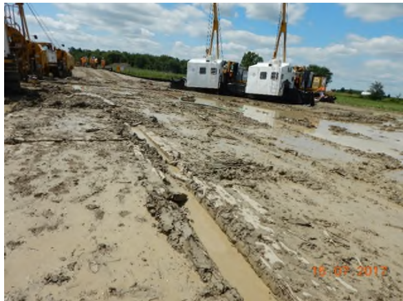
July 15 - P124 wood mats covered in mud and floating, ponded water and wet soil conditions
