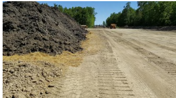
June 7 - P121 TLU area where topsoil from P122 woodlot stored on hay mulch layer
