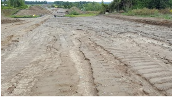
September 8 extensive subsoil rilling down slope indicative of susceptible erodible material
