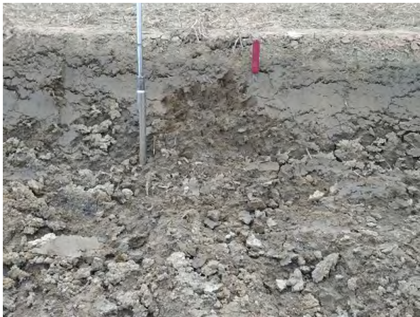
May 24 - P120 topsoil stripping depth exceeded for Brookston clay topsoil where 20cm adequate
