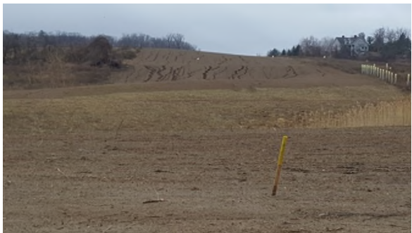
March 28 severe gully erosion overwinter looking west up slope
