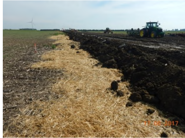
June 17 - P48 topsoil stripping piled onto straw mulch layer in TLU area along edge of easement
