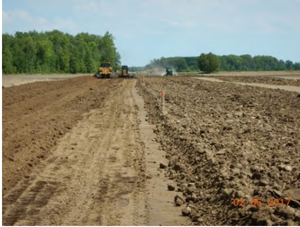
June 2 - P110 topsoil stripping sequence of discing, grader centre cut, bulldozer pushing windrow
