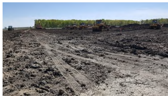
May 15 - P128 topsoil stripping using ten heavy machines done too early on moist clayey subsoils
