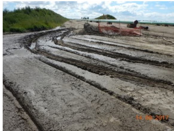
Sept 14 - P8 pickup truck tracks in wet saturated soil
