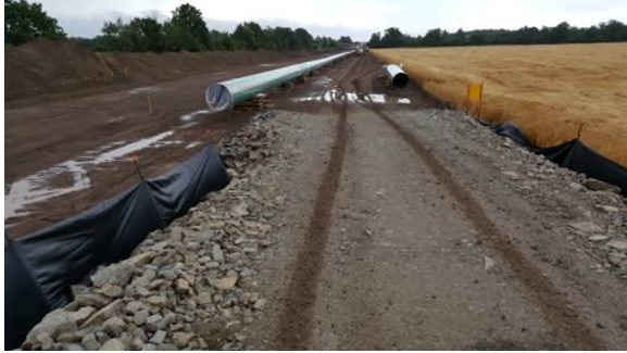
July 14 - HM44 pickup traffic on easement during wet soil shutdown
