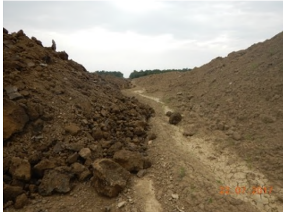
July 22 P121 some spoil materials occasionally piled onto topsoil seconds
