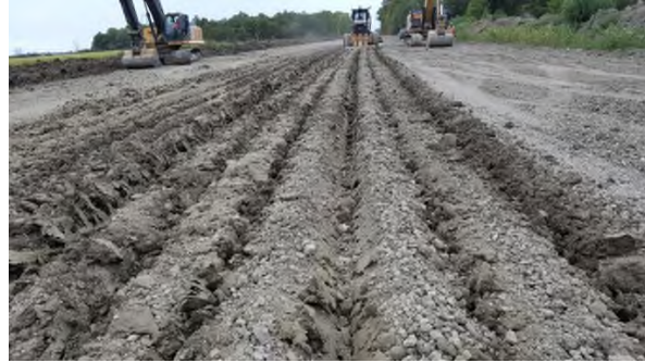
Sept 18 - P124 subsoil 'decompaction' in dry surface and moist clay subsurface conditions
