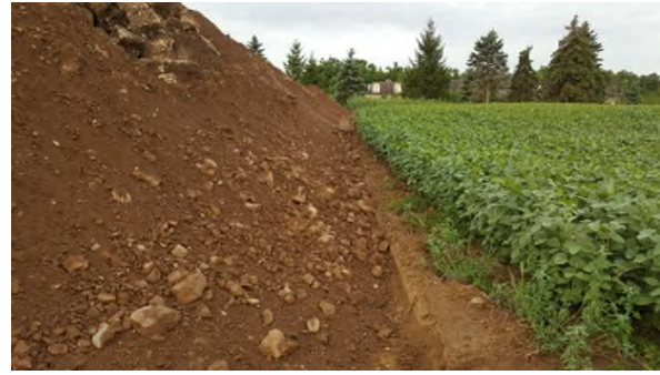
July 29 - HM28 subsoil pile exceeding TLU boundary encroaching into soybean crop
