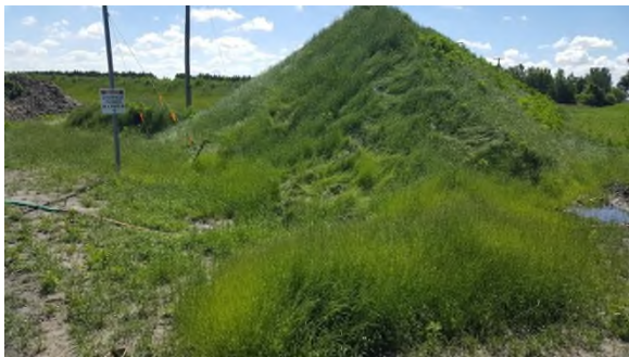
June 21 - P1 TLU topsoil pile hydroseeding well established for erosion protection
