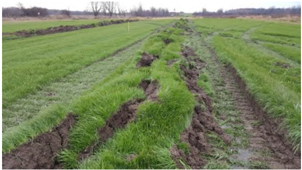
December 7 - HM44 tile installation trenches and topsoil rutting after completing in wet conditions
