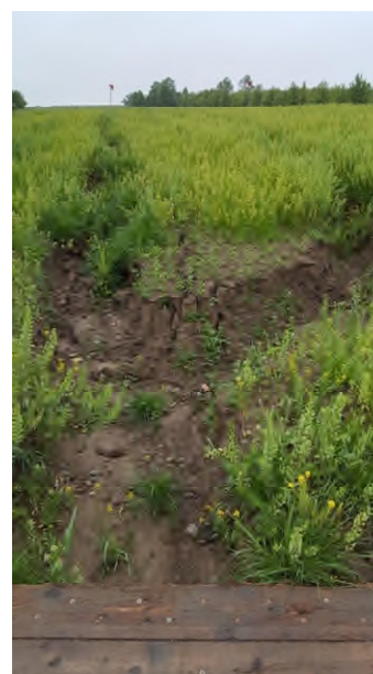
HM43 severe gully erosion on unprotected slope overwinter
