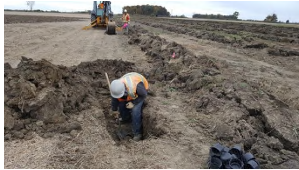
Oct 26 - P56 locating lateral tile, cutting and inserting drainage tile cap
