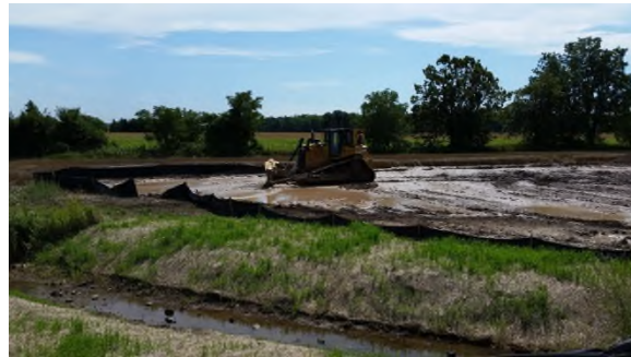
August 27 - HM44 bulldozer blading fully saturated soil to aid drying
