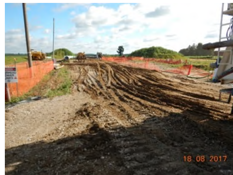
Aug 18 - P96 wet soils and ruts off the access ramp from hydrovac truck before mats installed
