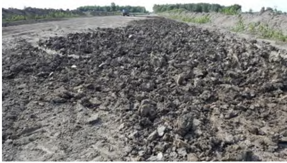
Sept 12 - P124 clay subsoil chiseled in wet areas intended to promote drying in good weather
