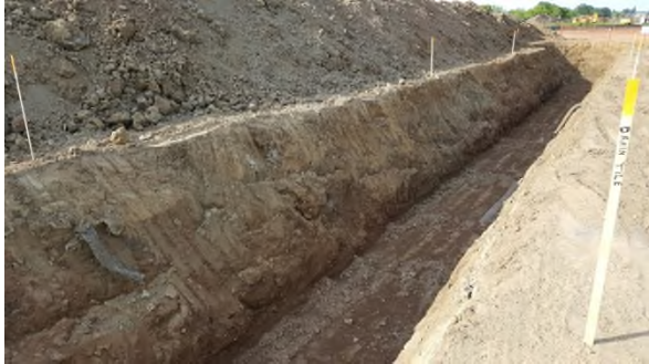
July 20 - HM45 drainage tile intercepted by trenching marked by wooden stakes
