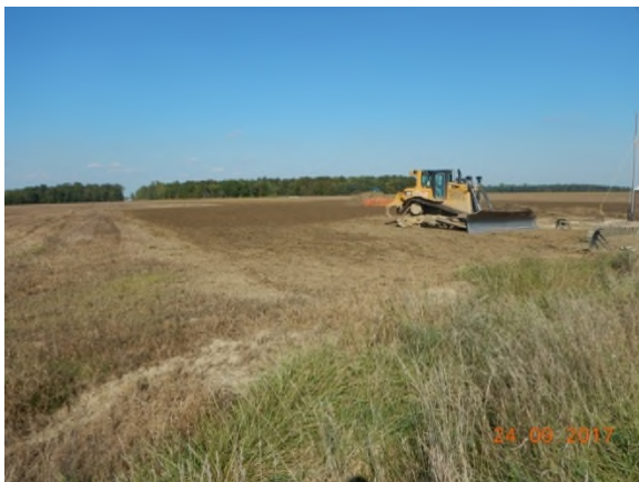
c) bulldozer spreading and grading topsoil
