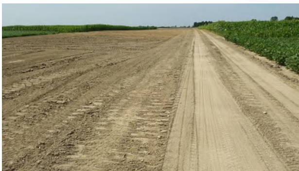
July 16 - P26 driving lane used for bridge removal compacting topsoil that had been returned
