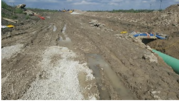
Sept 20 - P38 impact on subsoil from stream crossing activities under wet soil conditions
