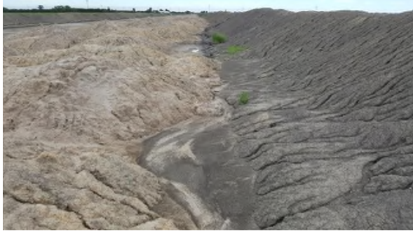
June 5 - P8 mixing of topsoil and extraneous subsoil piles overwinter with no separation
