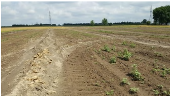
July 23 - P75 subsoil topsoil mixing from backhoe trenching used in locating lateral tiles
