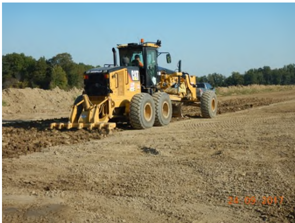
Sept 24 - P121 a) grader pulling ripper teeth decompacting subsoil to 30cm
