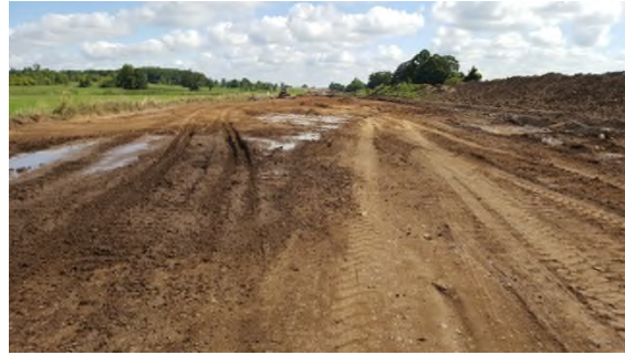
August 18 - HM39 tracks from some traffic on easement not avoiding wet soil
