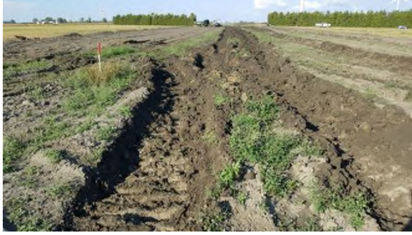
Oct 9 - P34 tile plow soil disturbance where tiles cutoff from trench to preconstruction header tile
