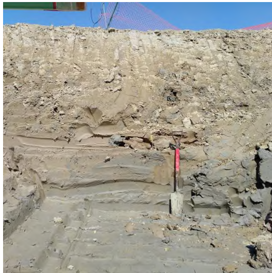
Aug 2 - P98 massive structured 'blue' clay subsoil exposed at 2.5m depth of trench`
