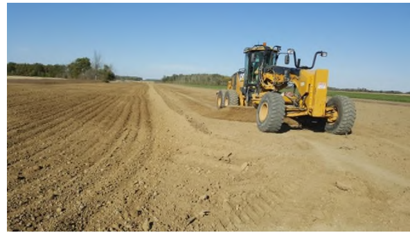
Oct 5 - P106 grader creating topsoil crown over trenchline
