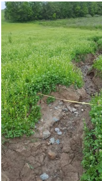
HM34 severe gully erosion (4ft.) on bare unprotected slope overwinter
