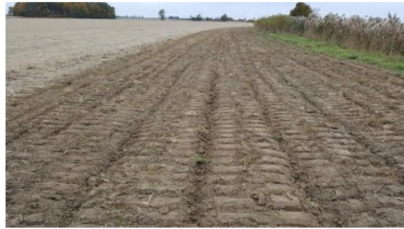
Oct 26 - P55 partial decompaction of access laneway to easement using only parallel passes
