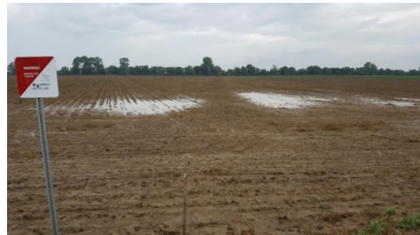
July 24 - P94 ponded water beside trench crown of fall restored and released property
