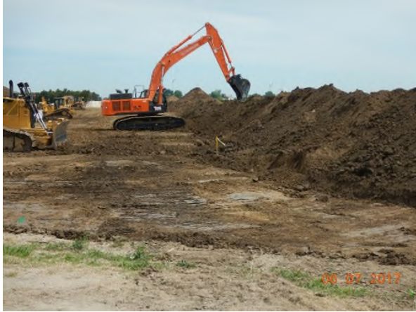
July 6 - P24 topsoil that spilled over the back of pile off easement being pulled back onto pile
