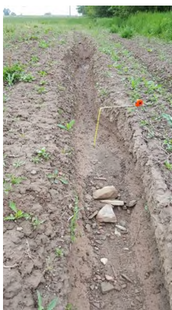
HM40 deep rill erosion formed from flow across easement
