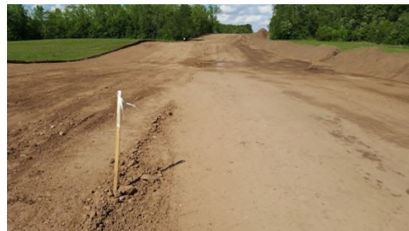
June 6 - HM14 topsoil stripped across easement and stored in one pile
