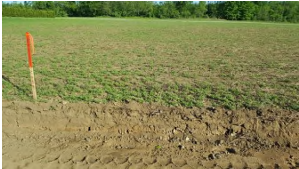
May 30 - HM13 topsoil A horizon (darker) and B horizon (reddish) stripped together
