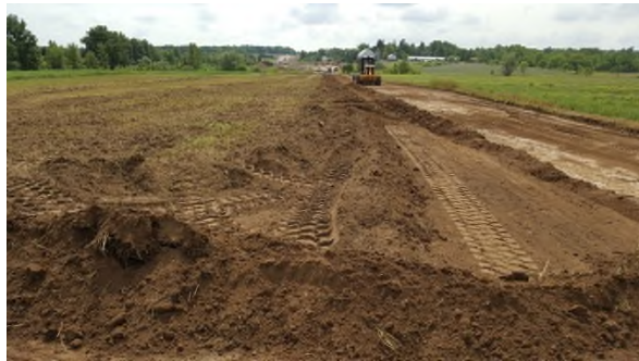
August 15 - HM36 grader initiates topsoil stripping to determine proper depth
