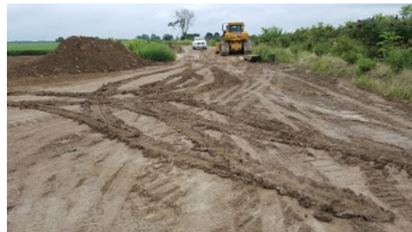
Aug 1/18 - P56 pickup turnaround tracks on wet soil just beyond mat lane
