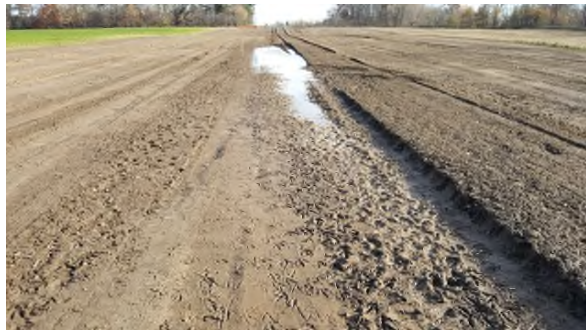
December 1 - HM36 trenchline mound of replaced topsoil trapping surface water flow
