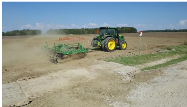
d) cultivator leveling topsoil (Sept 26)
