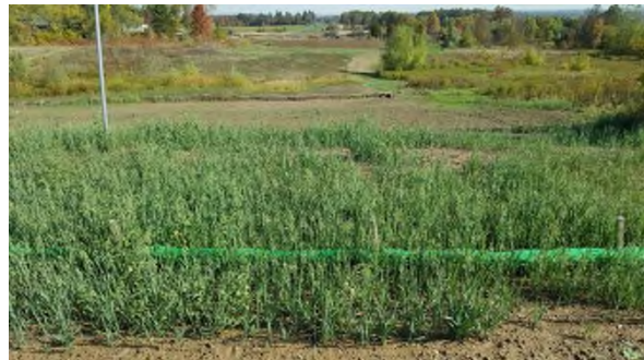
October 10 established additional erosion protection across foot slope done on August 21
