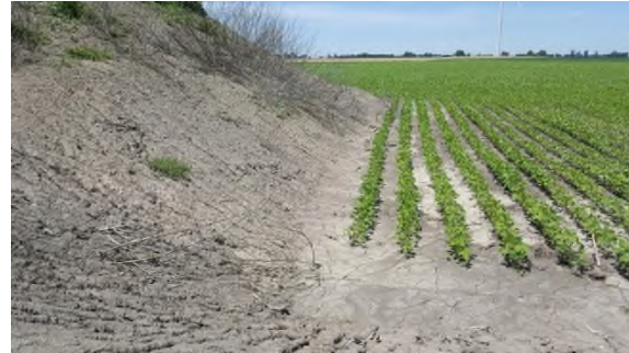
June 26 - P61 large topsoil pile in TLU has eroded sediment without containment into adjacent field
