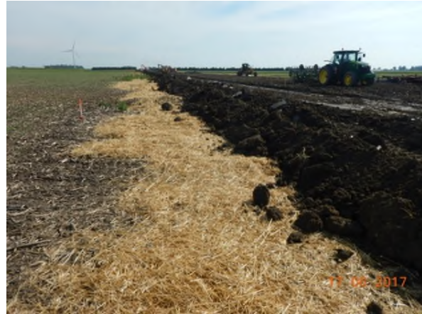
June 17 - P48 topsoil stripping piled onto straw mulch layer in TLU area along edge of easement
