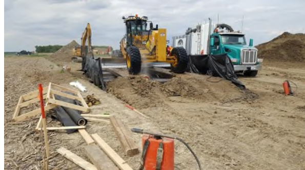
May 23 - P98 wash station cleaning infected SCN topsoil from machinery adjacent to non SCN field
