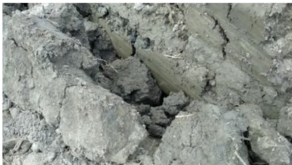
Sept 19 - P106 smearing effect affecting drainage when tile installed into moist, plastic clayey soil
