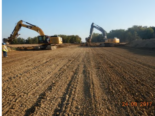
b) excavators pulling topsoil piles onto decompacted and levelled subsoil
