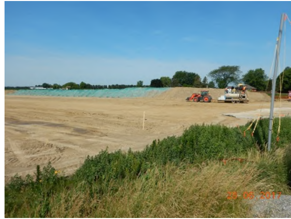
June 29 - P72 hydroseed spraying of topsoil piles in TLU of annual ryegrass on sandy soils
