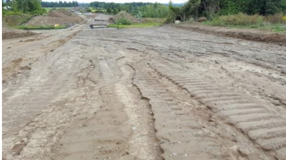
September 8 extensive subsoil rilling down slope indicative of susceptible erodible material
