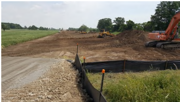
June 20 - HM39 topsoil stripping being completed by multiple operators
