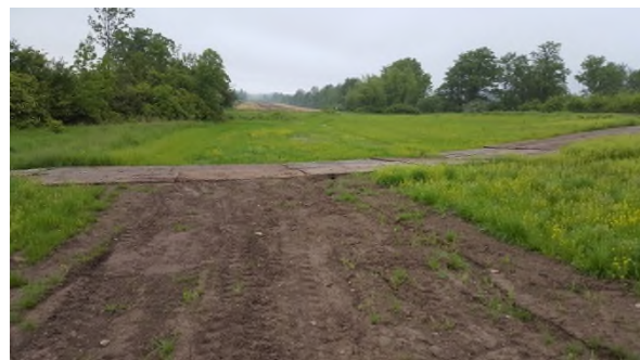
HM43 wood mat access provided across easement in spring after rutting and erosion - June 5
