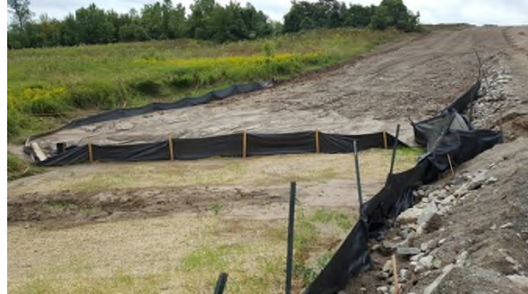
September 8 subsoil sediment deposition at toe slope from water erosion adjacent to creek
