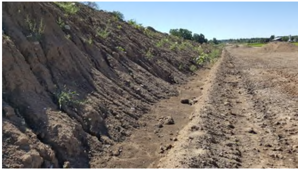
September 12 - HM40 topsoil pile eroded sediment captured by transition layer pile
