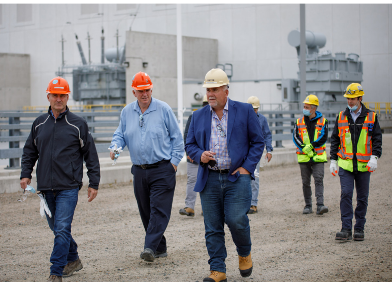
Minister of Energy Todd Smith tours the Smoky Falls Generating Station located on the Mattagami River near Kapuskasing. Smoky Falls Generating Station is operated by OPG in partnership with Moose Cree First Nation and has been in service since 1931 with a capacity of 267 MW.
