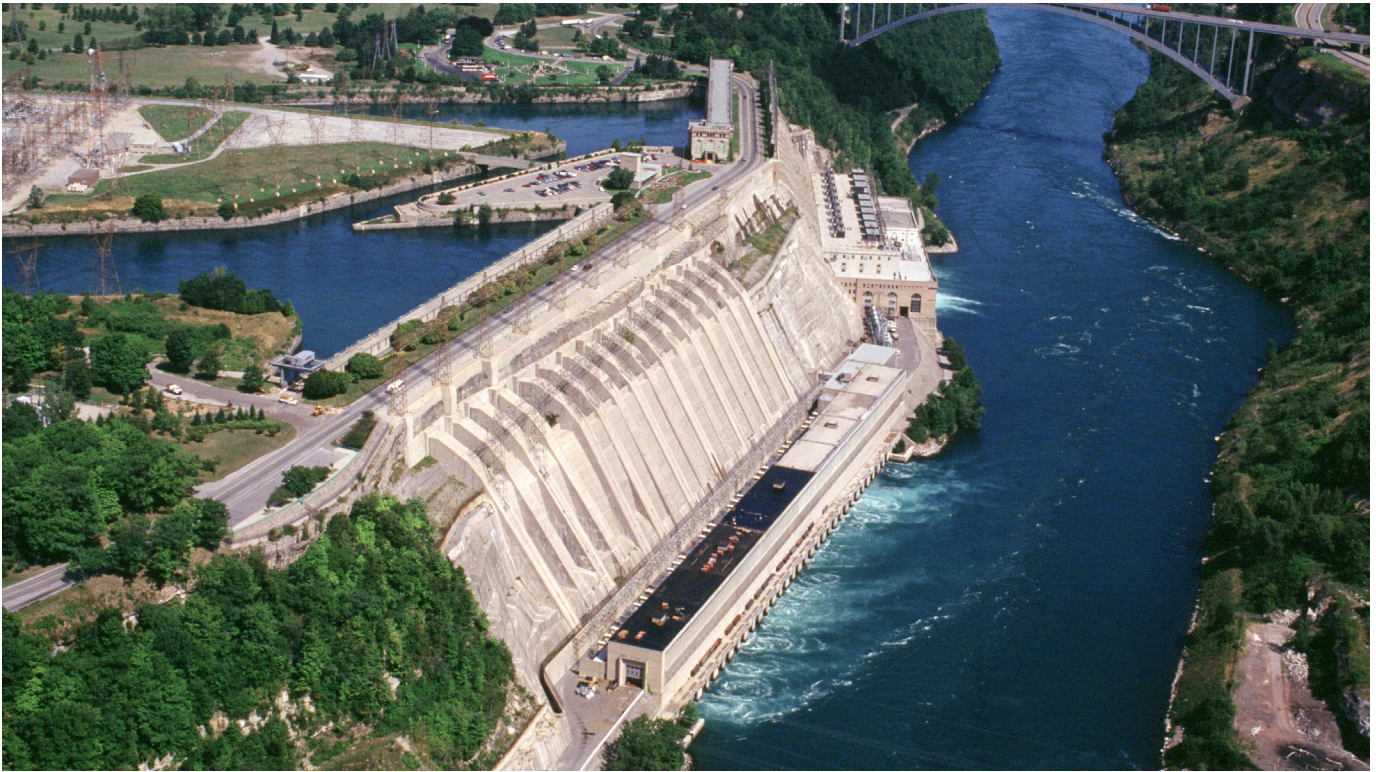
Sir Adam Beck Hydroelectric Generating Station.
