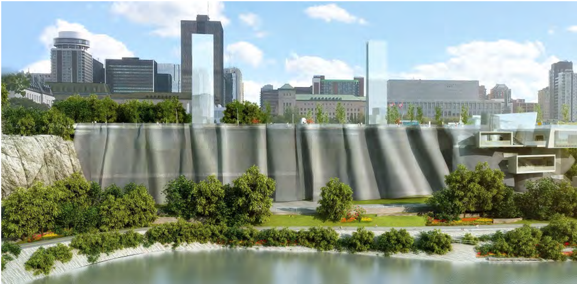
View of the Cliff plant from Gatineau showing the exterior and the stainless steel stacks.
