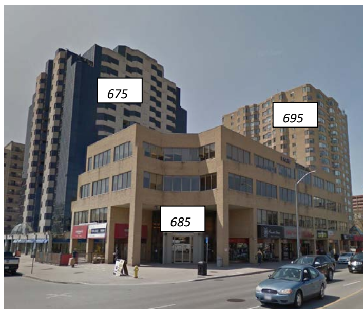
Customer Substation CS 315: 675, 685 & 695 Richmond St.
