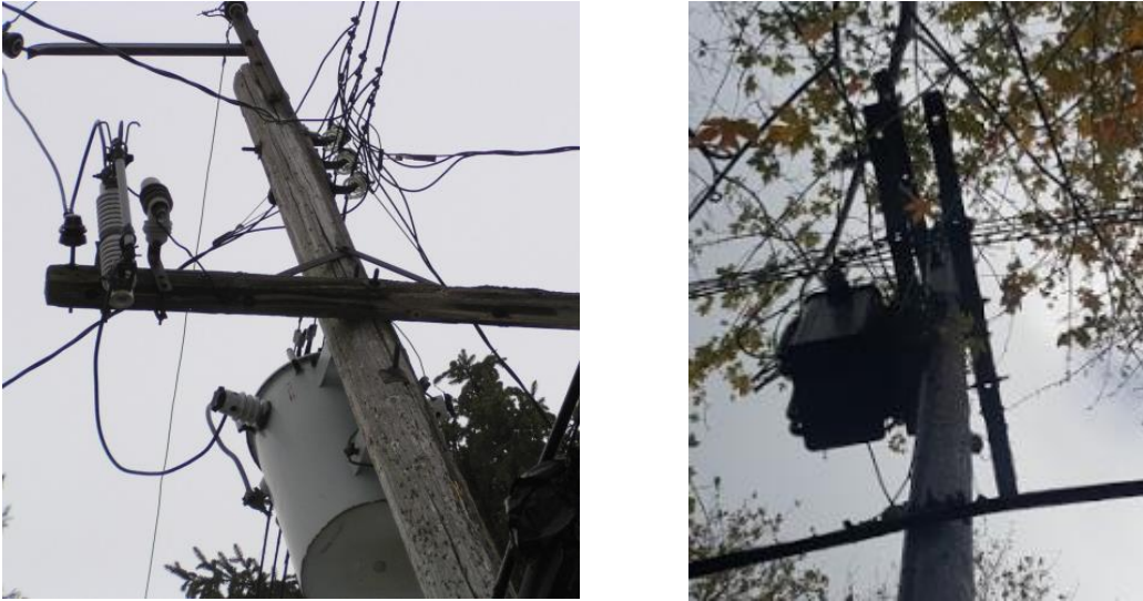
Figure 22: Rear Lot Plant Condition
