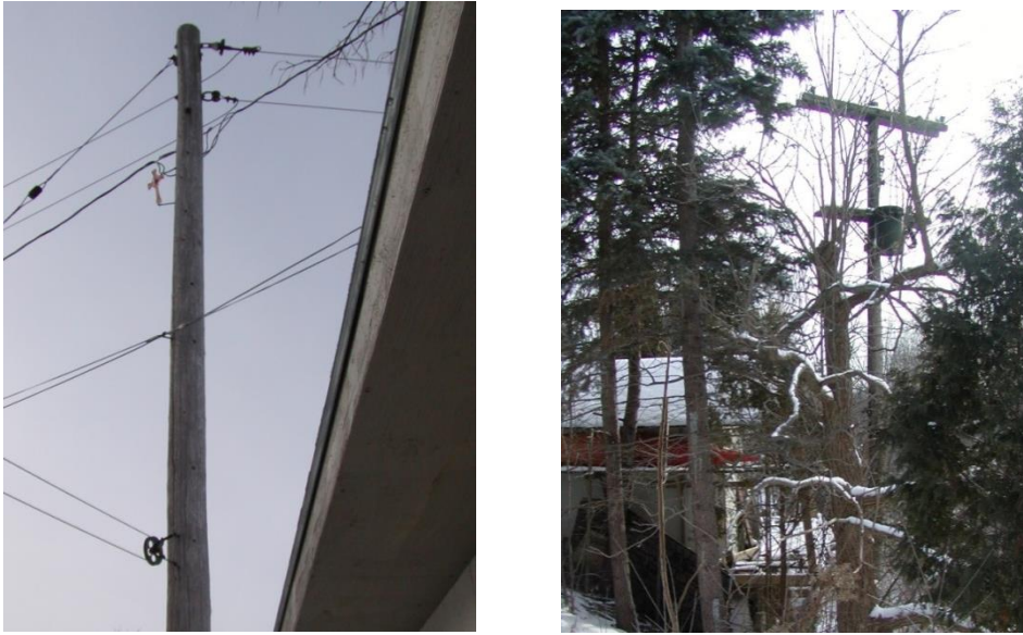
Figure 25: Close proximity of the equipment to the buildings
