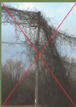
Guy-wire growth contacting electrical equipment & powerlines
