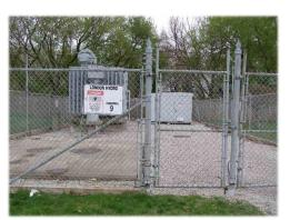
Outdoor Metal-clad Substation
