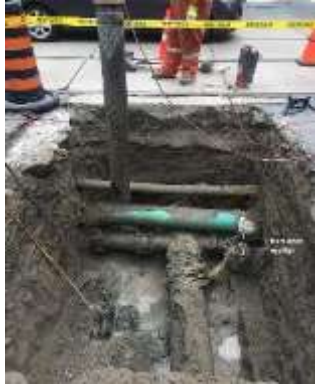
Figure 5.2-15: Leak investigation on vintage NPS 12 gas main
