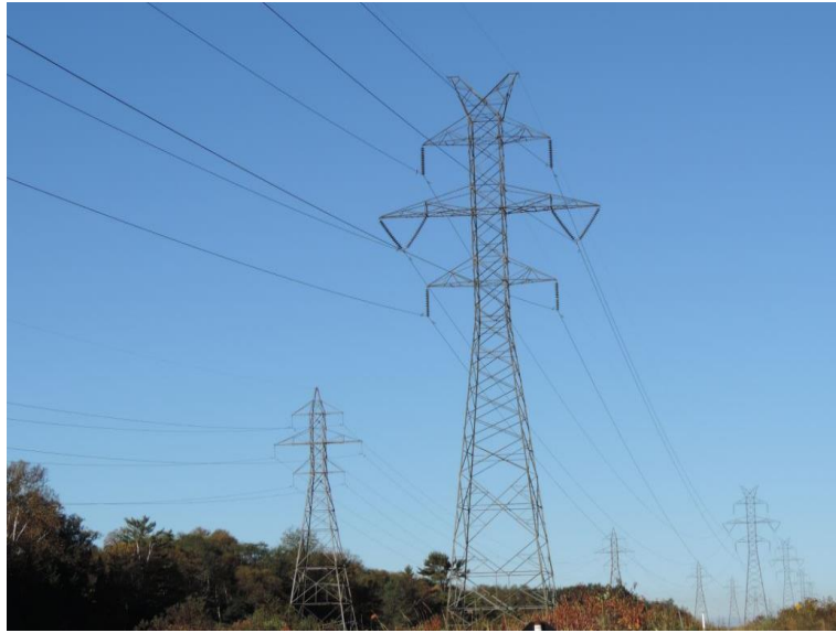
Figure 4-2: Lattice Towers near Third Line TS
