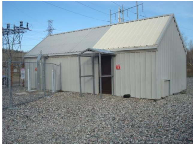
Figure 3-2: Anjigami TS Control Building
