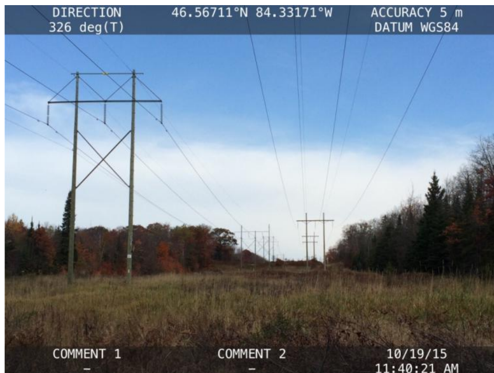
Figure 1-1: K24G and No.3 Sault at Fourth Line Crossing
