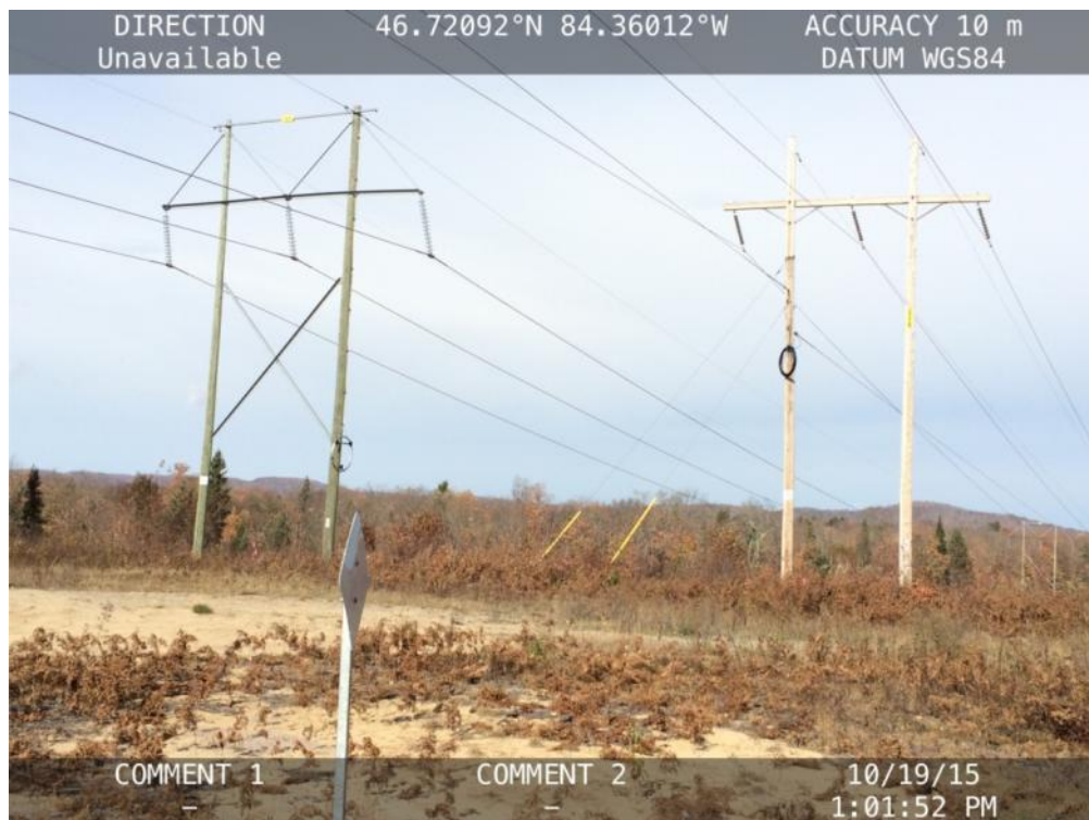
Figure 3-1: No.3 Sault Structure (Towards Right)
