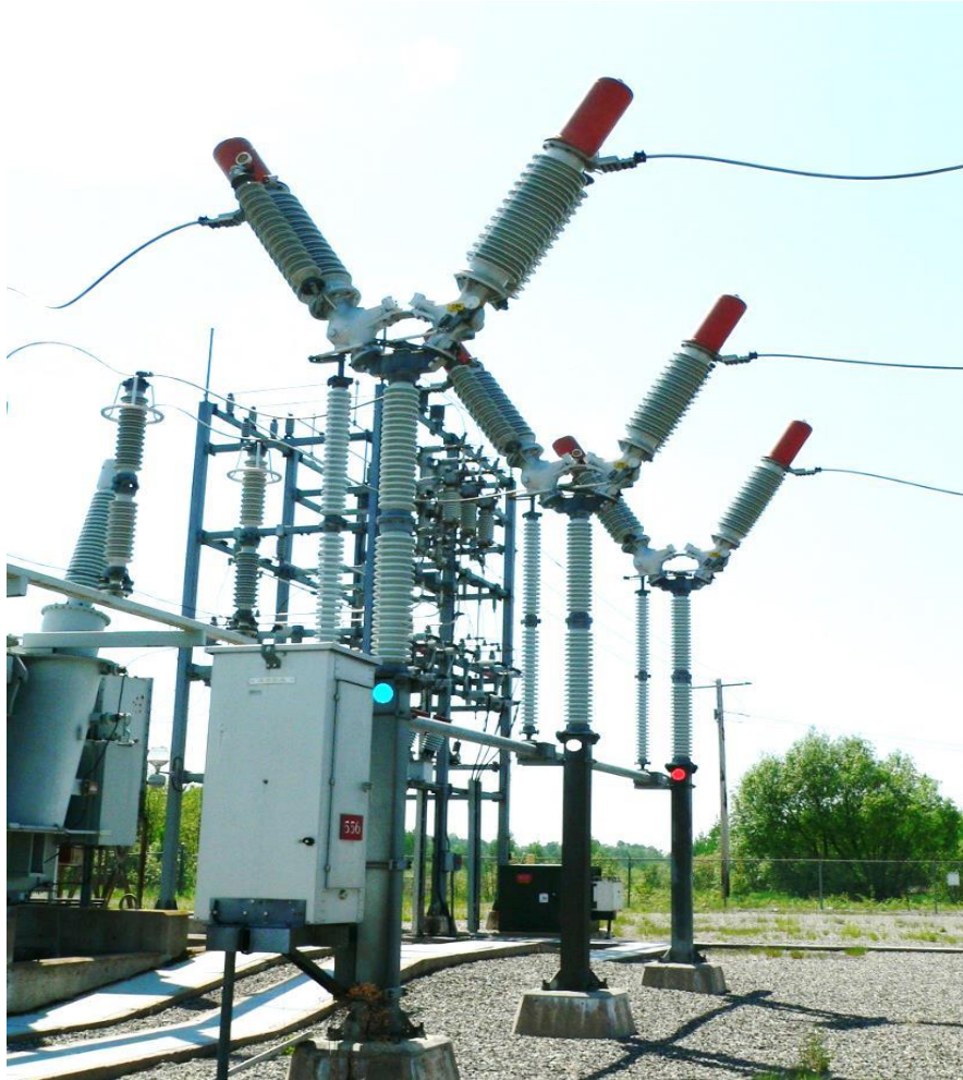
Figure 11 – CB 556 Minimum Oil Breaker at Echo River TS
