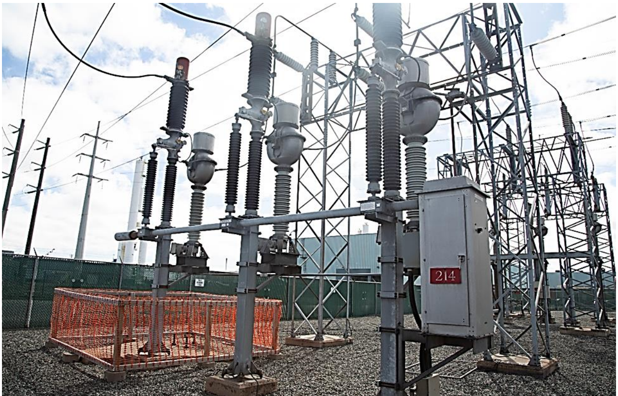
Figure 16 – Existing Minimum Oil Circuit Breaker 214 at Steelton TS
