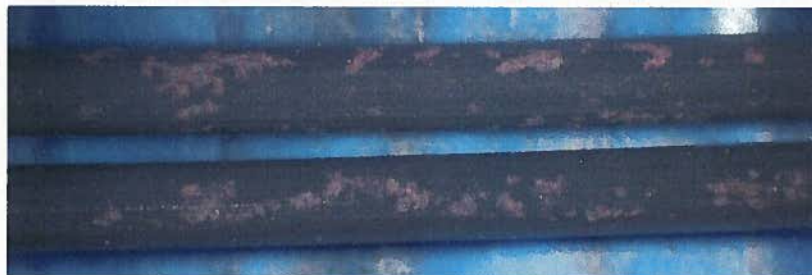
Figure 8d - Steel Wires - Outer Surface of Two Wires after Removing Zinc
