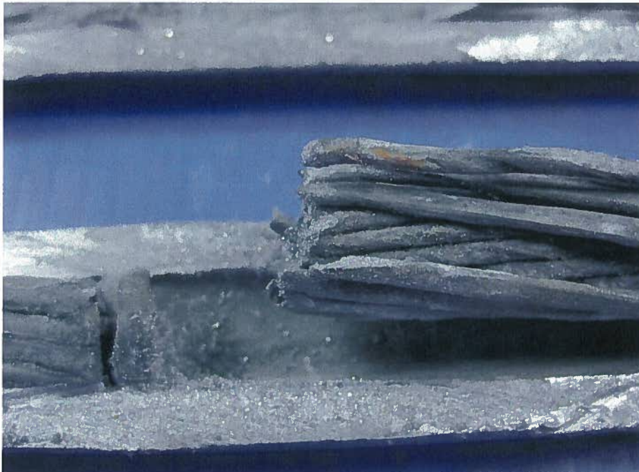
Figure 23: Dissected Connector: note onset of corrosion on conductor strands (right-hand)
