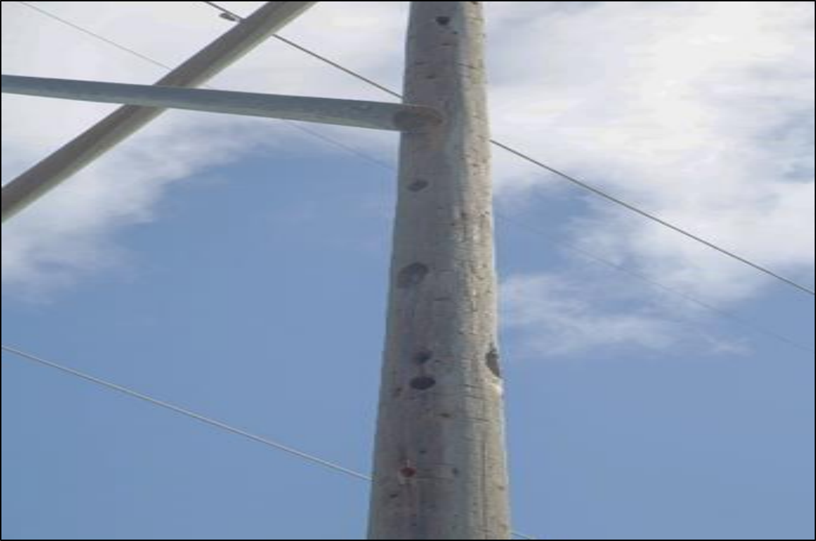
Figure 1 – Circuit P22G Structure with Extensive Woodpecker Damage
