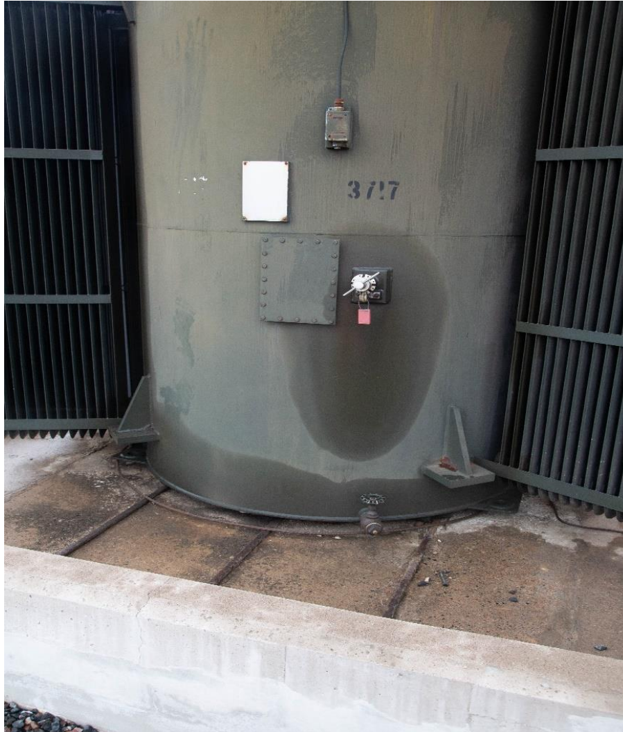
Figure 15 – Evidence of Extensive Transformer Oil Leaking at Goulais TS
