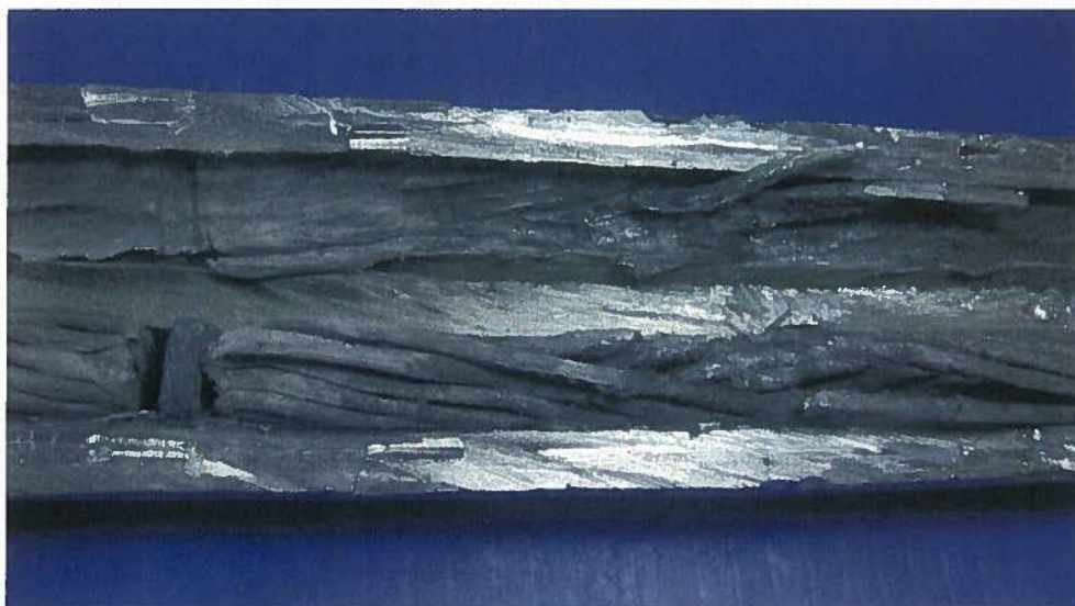
Figure 19: Dissected Connector: possible conductor damage (one area) due to overheating or due to prep work during installation
