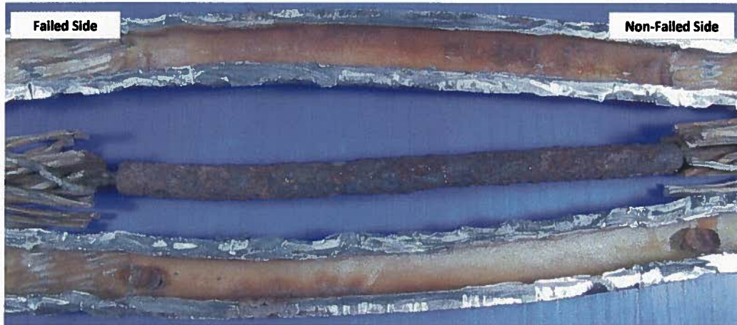
Figure 6 - Steel Wires Inside Splice
