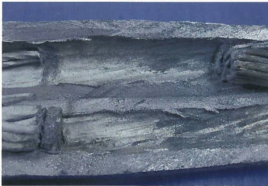
Figure 7: Failed Connector: imprints on connector sleeve point to proper conductor insertion during installation and conductor partial withdrawal during overheating and failure
