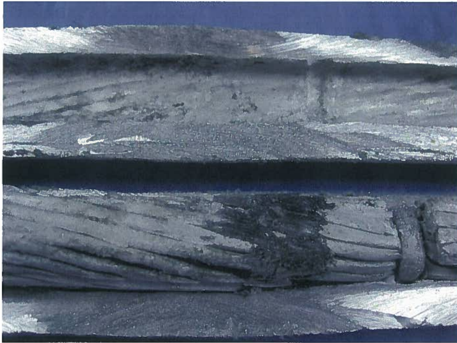
Figure 12: Dissected Connector: note electrical tape left on conductor during installation – reduced electrical contact inside connector
