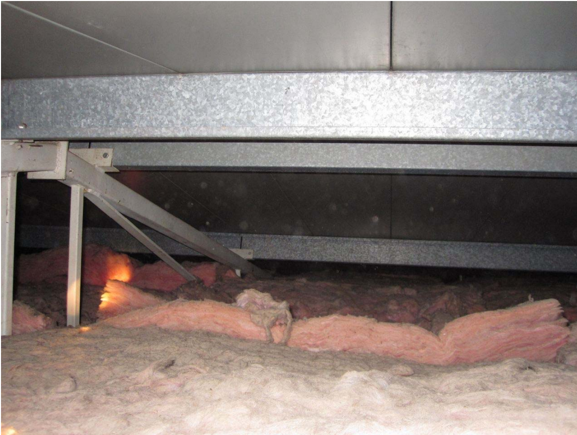
Photo#13 – Roof Panel Support/Insulation (Big Trout Lake)
