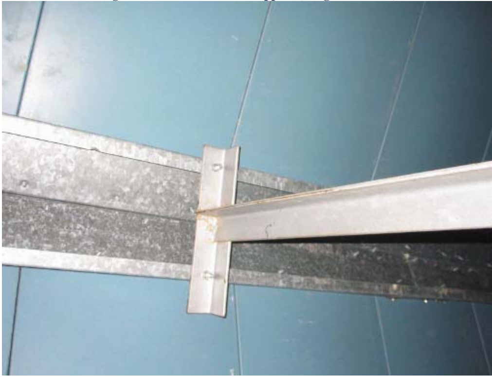
Figure 5: Roof Panel Peak Support (Kingfisher Lake)
