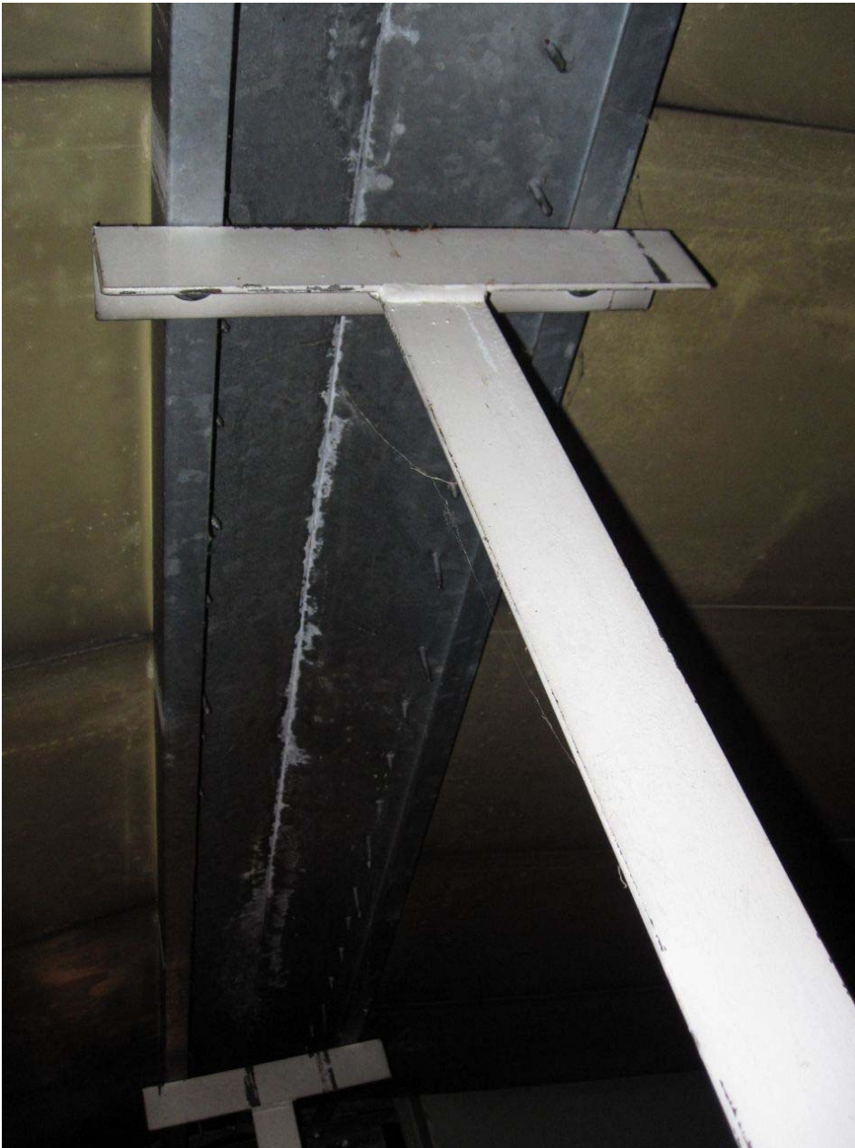
Photo#8 – Roof Panel Peak Support Framing (Lansdowne House)
