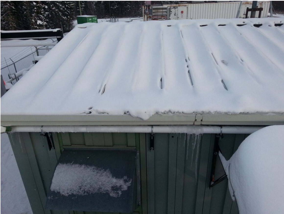
Photo#16 – Beginnings of Visible Ice Formation (Weagamow)
