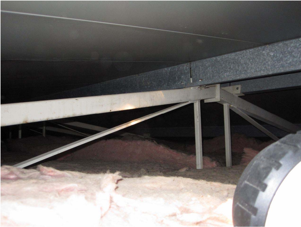
Photo#11 – Roof Framing (Big Trout Lake)
