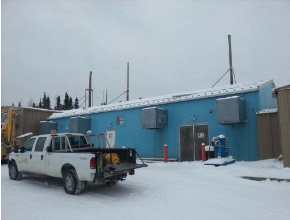
Figure 1: Kingfisher Lake Diesel Generating Station (Exterior)
