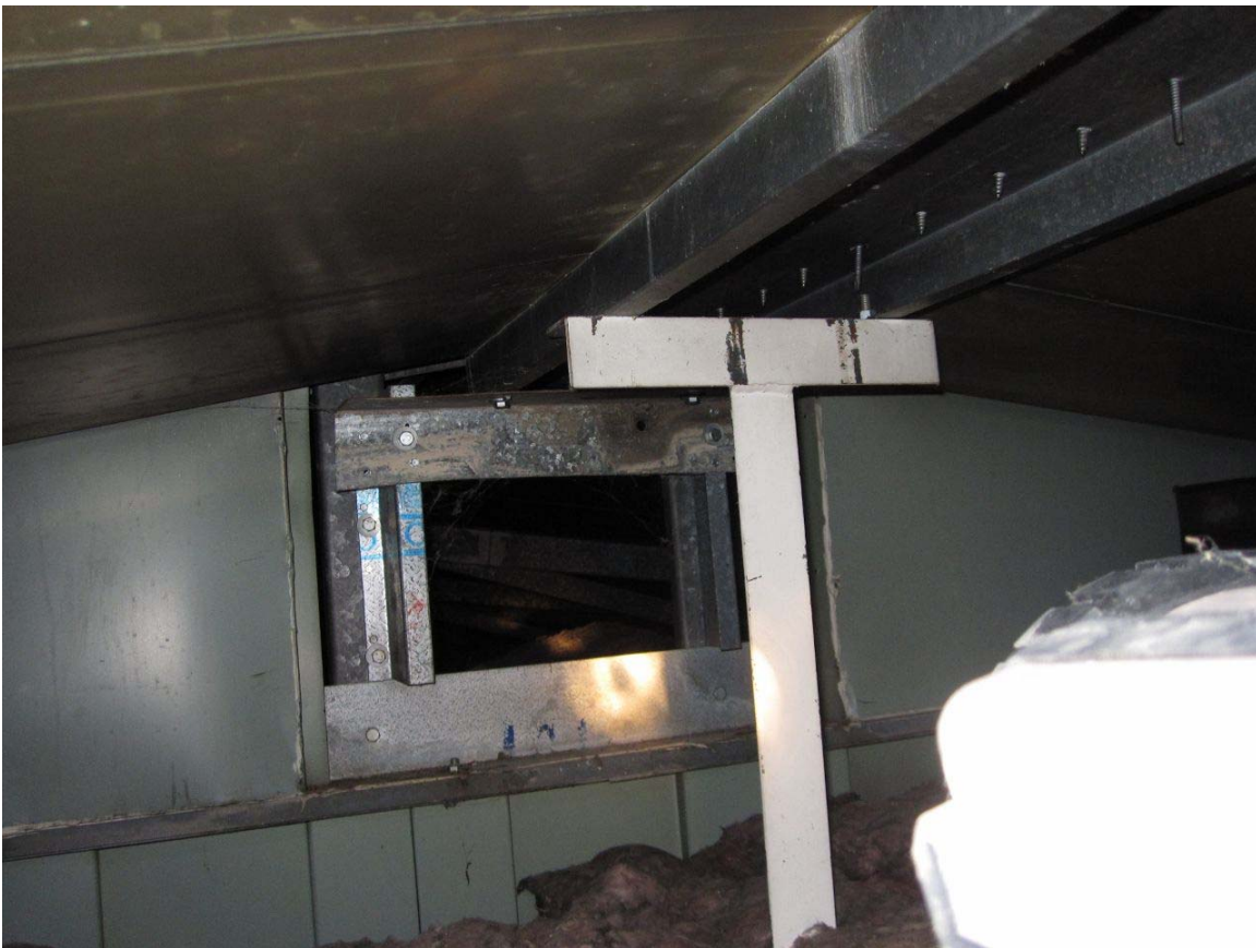
Photo#10 – Roof Construction Transition (Lansdowne House)
