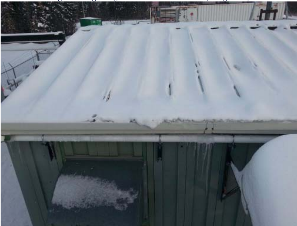
Figure 9: Beginnings of Visible Ice Formation (Weagamow)
