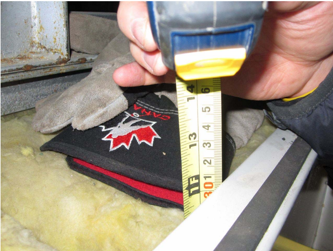
Photo#2 – Existing Roof Insulation Thickness (Kingfisher Lake)
