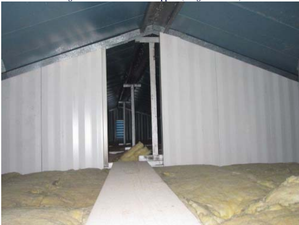
Figure 5: Roof Panel Peak Support (Kingfisher Lake)
