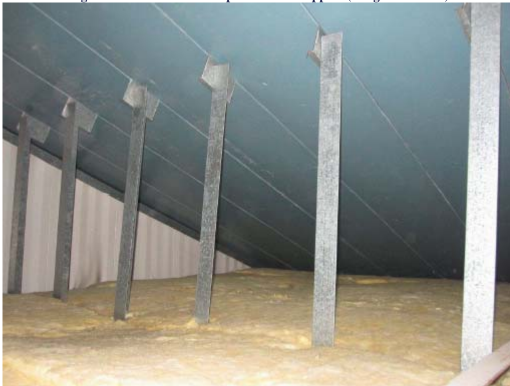
Figure 3: Roof Panel Mid-Span & Eave Support (Kingfisher Lake)
