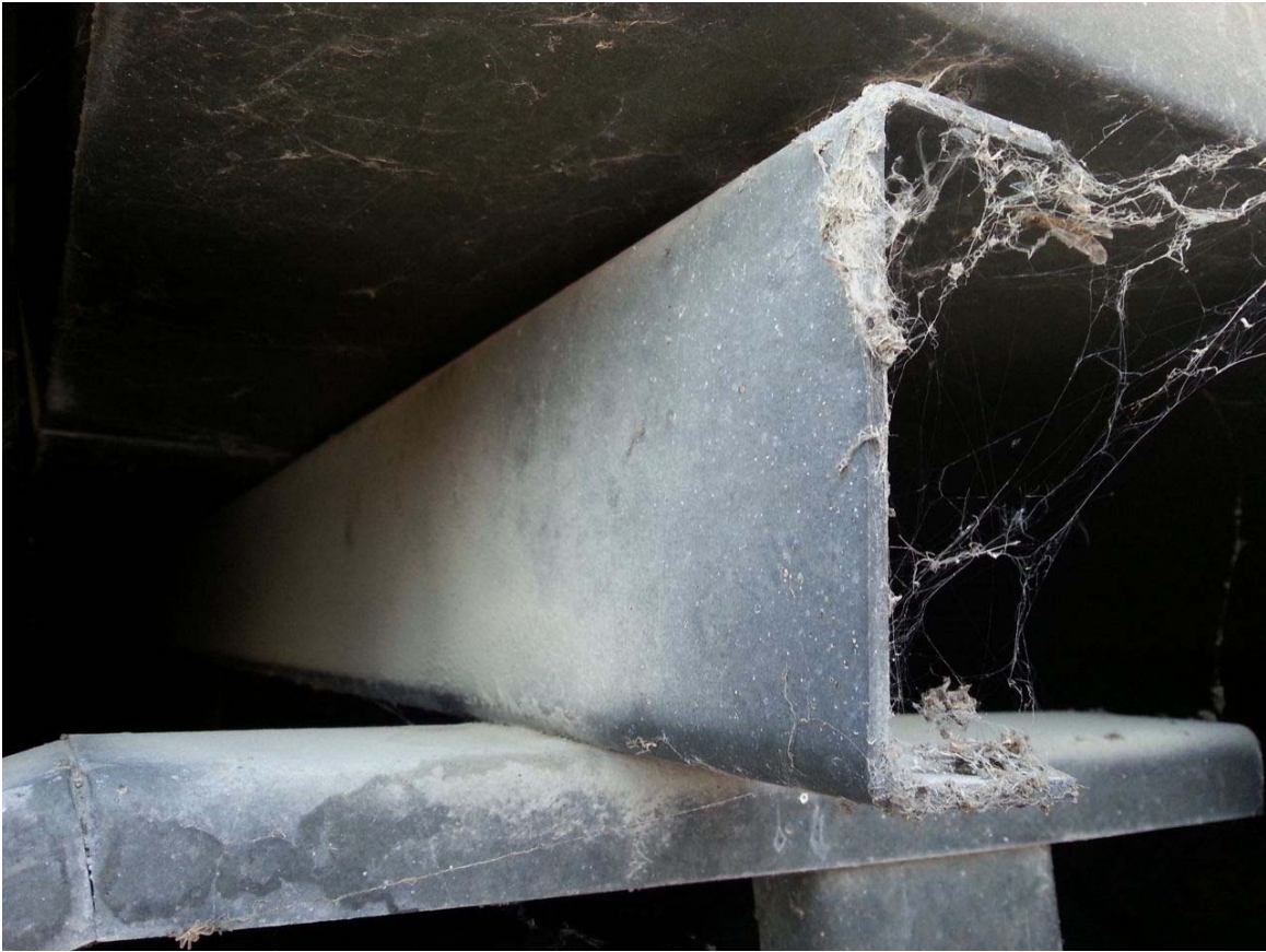
Photo#15 – CFC Purlins (Weagamow)
