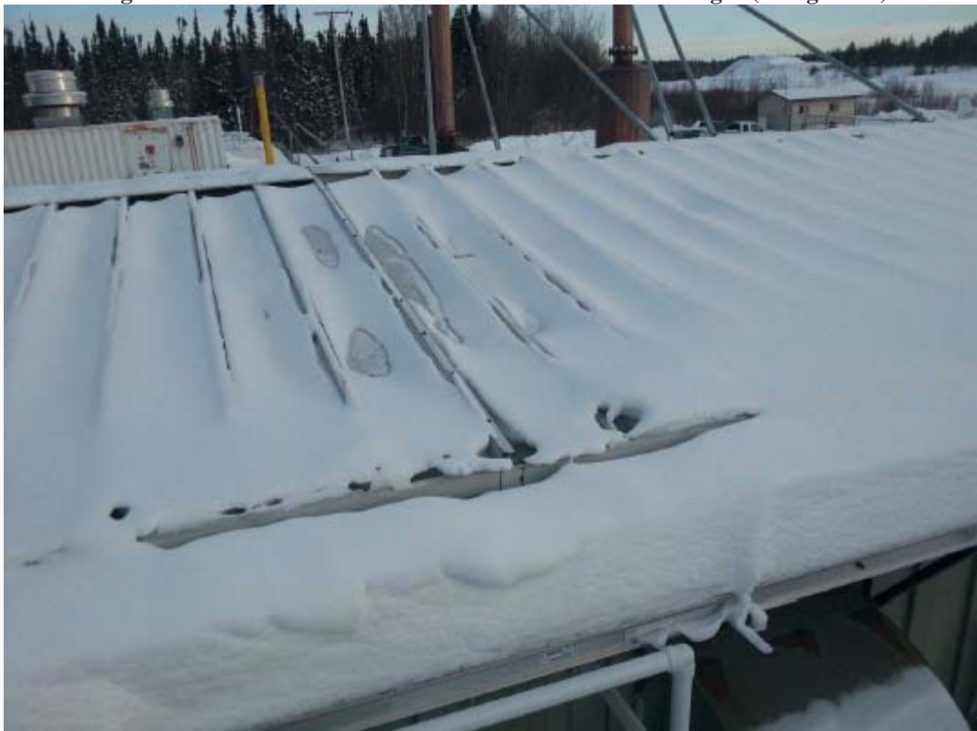
Figure 11: Visible Heat Loss & Roof Panel Deterioration Signs (Weagamow)
