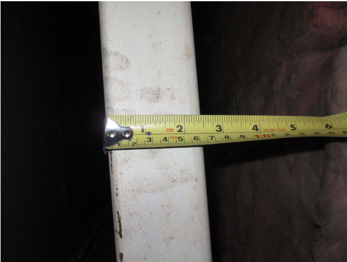
Photo#12 – Roof Truss Top Chord (Big Trout Lake)
