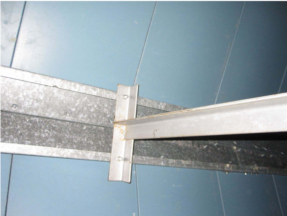
Photo#4 – Roof Panel Peak Support (Kingfisher Lake)
