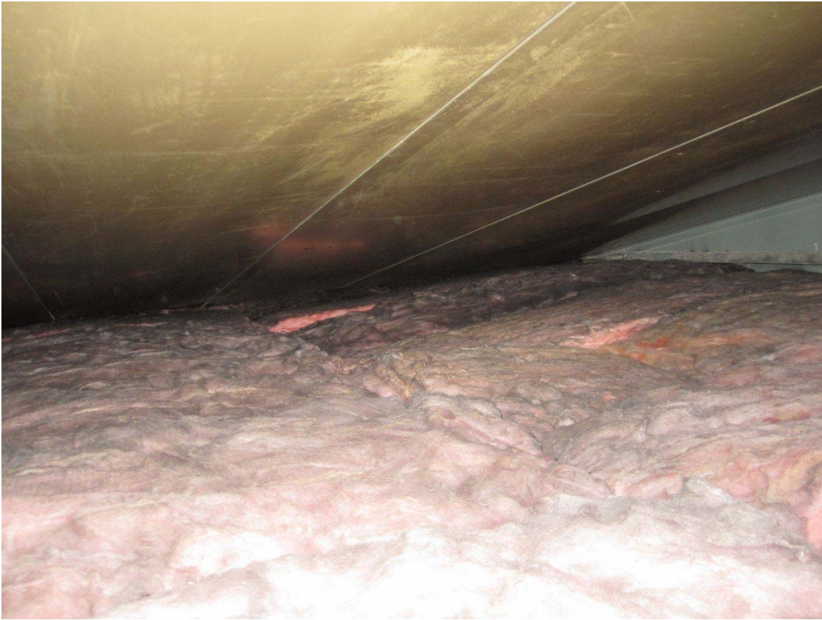
Photo#9 – Roof Panel Eave Support/Insulation (Lansdowne House)
