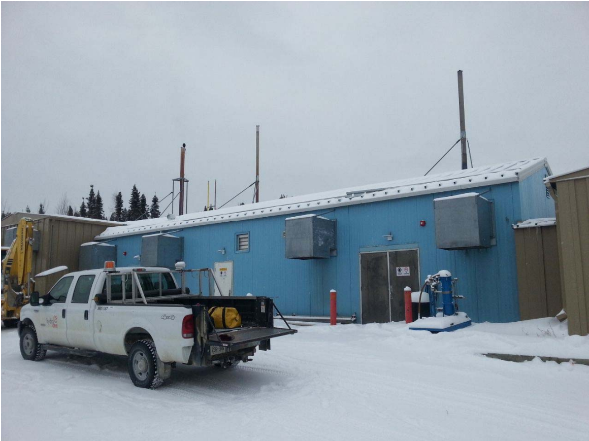
Photo#1 – Kingfisher Lake Diesel Generator Station (Exterior)
