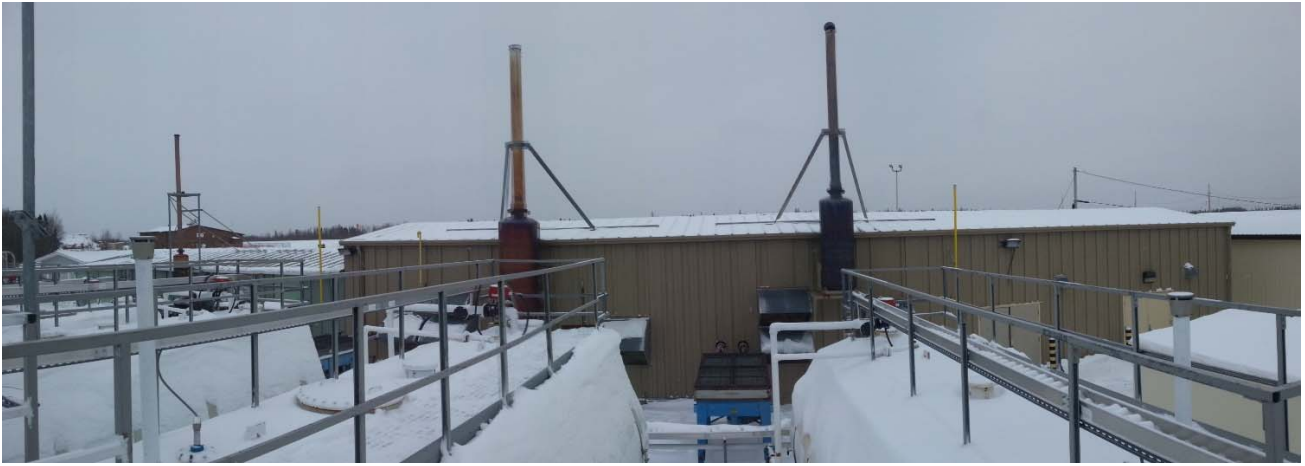
Photo#7 – Existing Roof Elevation Transition (Lansdowne House)
