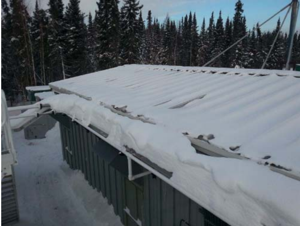
Figure 11: Visible Heat Loss & Roof Panel Deterioration Signs (Weagamow)
