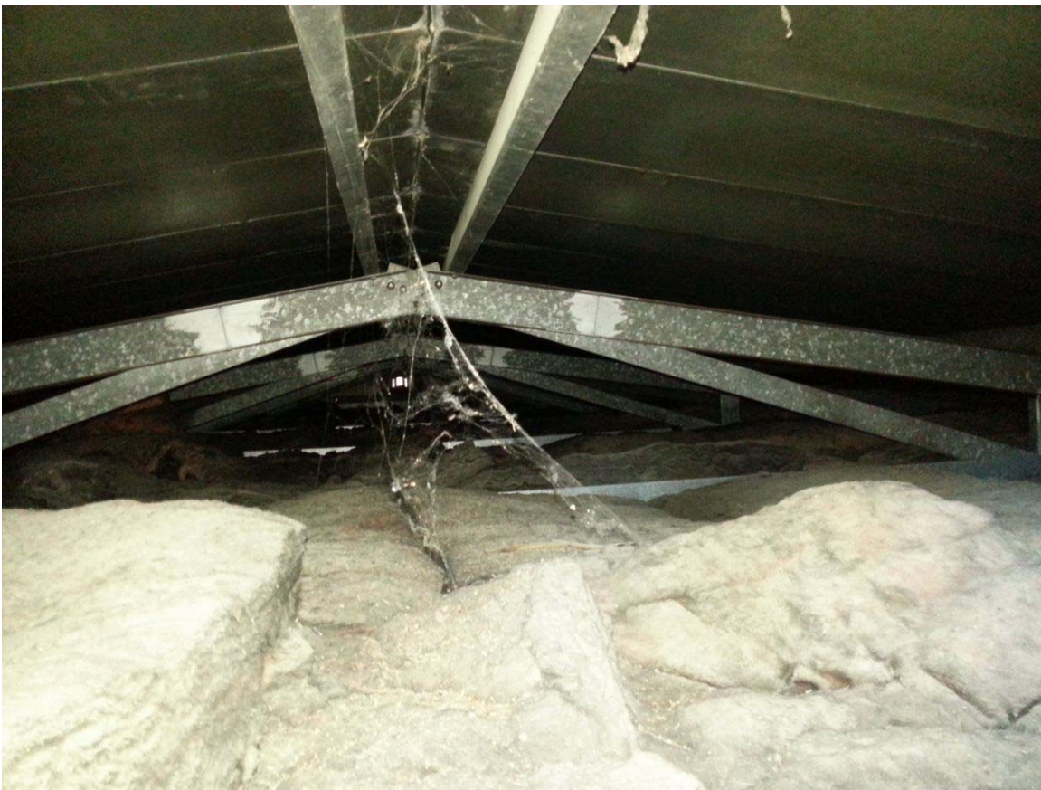
Photo#14 – Roof Framing (Weagamow)
