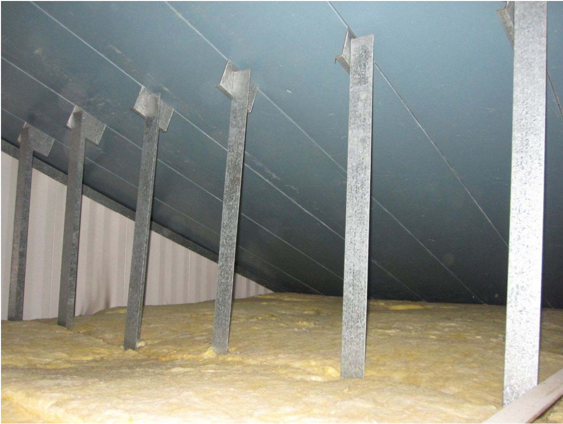
Photo#3 – Roof Panel Mid-Span & Eave Support (Kingfisher Lake)
