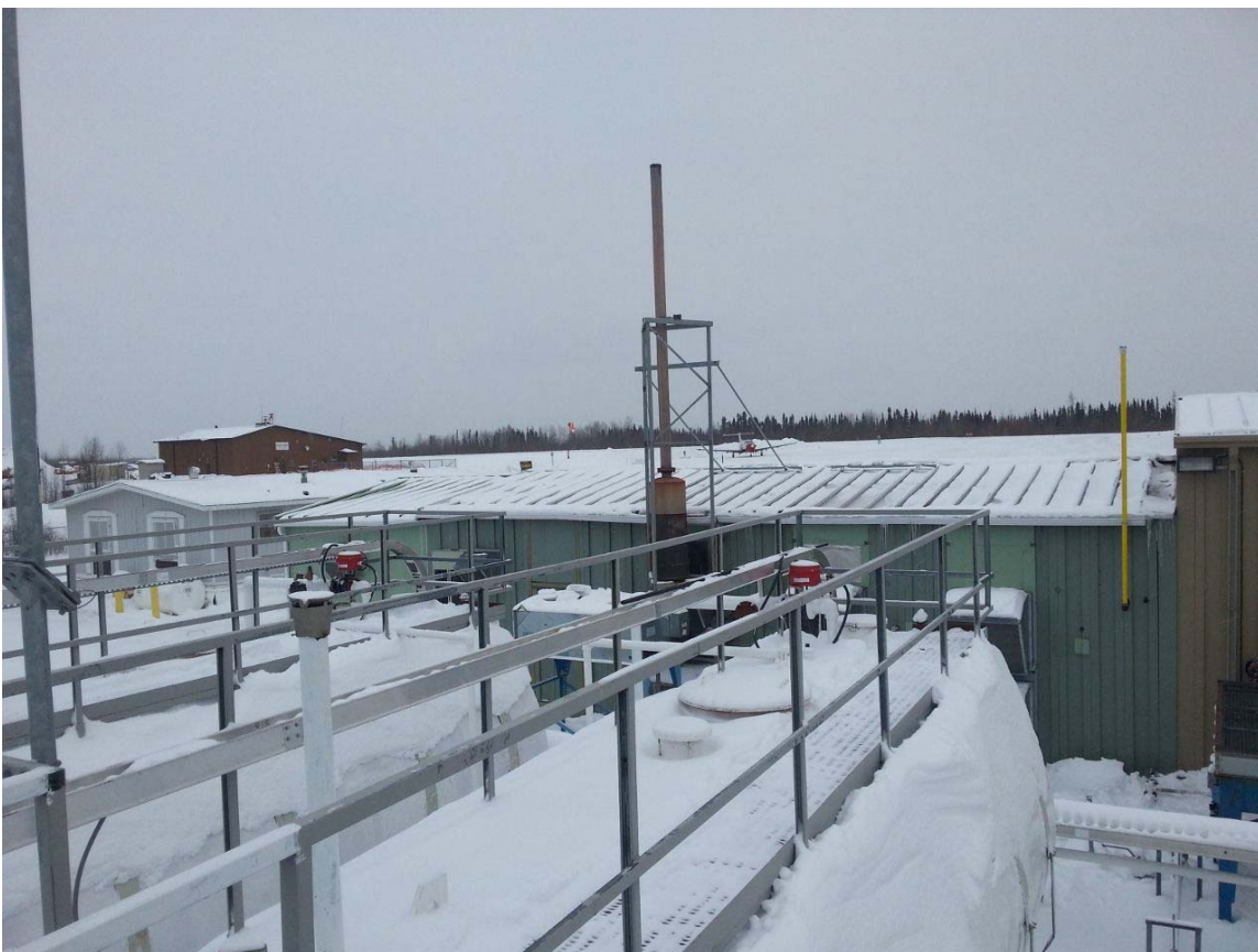
Photo#6 – Lansdowne House Diesel Generator Station(Exterior)
