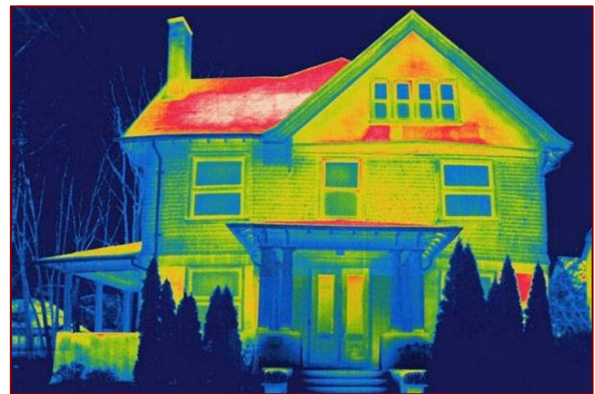
Figure 11-2, Application of Infrared Imagery to Highlight Household Leaks
