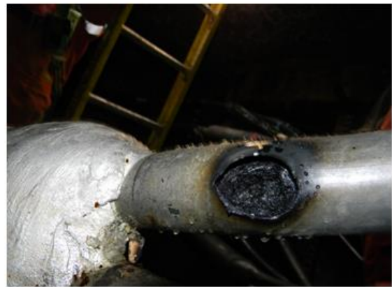
Faulted Cable
