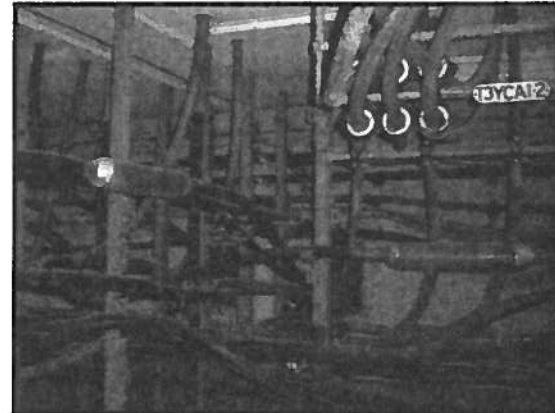
Figure 3: Windsor Station Cable Congestion
