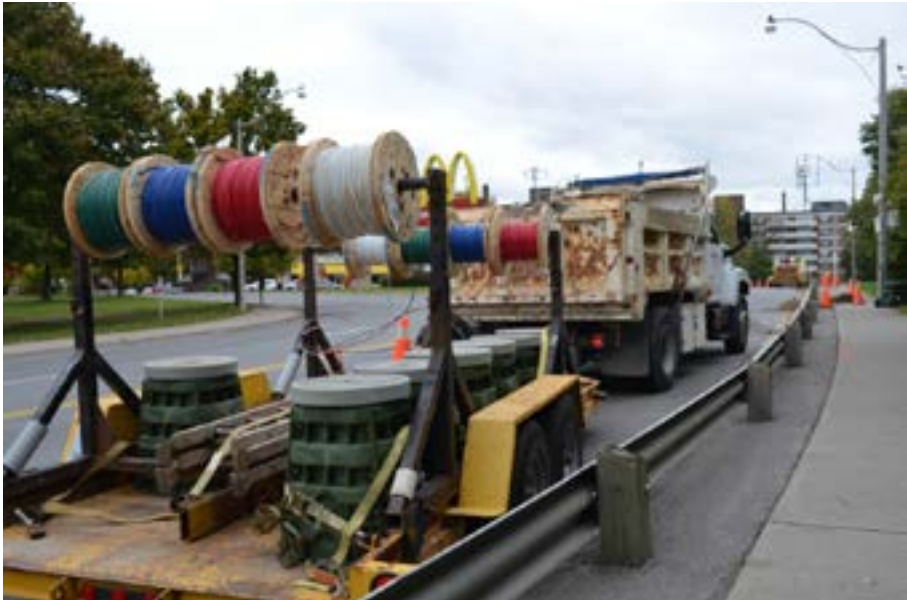
Crew working on installations
