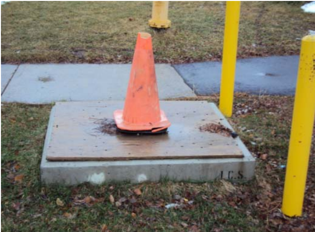
1 Figure 16: Civil work that has been completed in the Rexdale Colony rear lot area, awaiting 2 electrical installation (photo taken in 2012)
