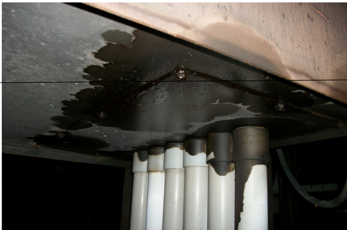
Figure 20: Circuit Breaker at Bathurst TS 85M1 (February 2, 2012)
