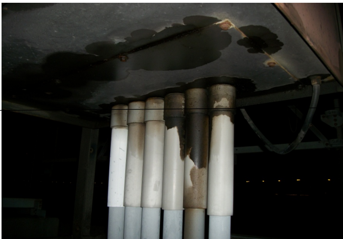
Figure 22: Circuit Breaker at Bathurst TS 85M2 (February 2, 2012)
