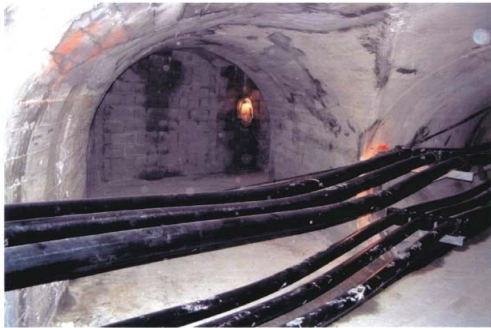
Figure 2 Existing break out at HONI transmission tunnel for Bremner TS tunnel
