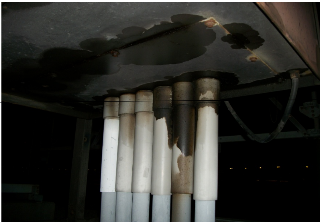
Figure 22: Circuit Breaker at Bathurst TS 85M2 (February 2, 2012)
