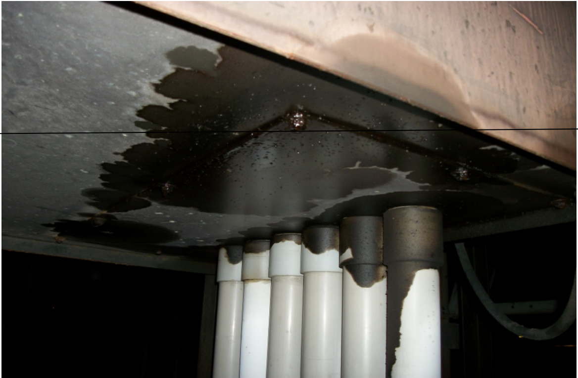
Figure 20: Circuit Breaker at Bathurst TS 85M1 (February 2, 2012)
