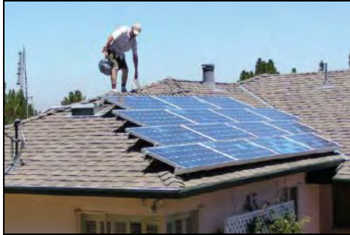
Figure 3-11 Residential Rooftop Photovoltaic Panels (Source: NREL)
