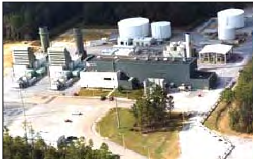
Figure 4-6 Aerial View of an underground CAES plant in McIntosh, Alabama, one of two such facilities operating in the world. The other is in Huntorf, Germany.
