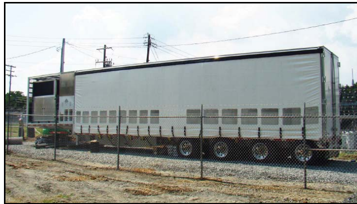
Figure ES-4 Premium Power's 0.5-MW/2.8 MWh TransFlow 2000 Transportable Zinc-Bromine Energy Storage System Preparing for Demonstration by EPRI.
