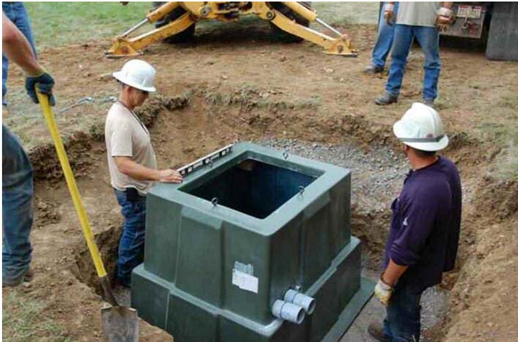
Figure H-1. Installing Below Ground Battery Vault – 25 kW AEP CES
