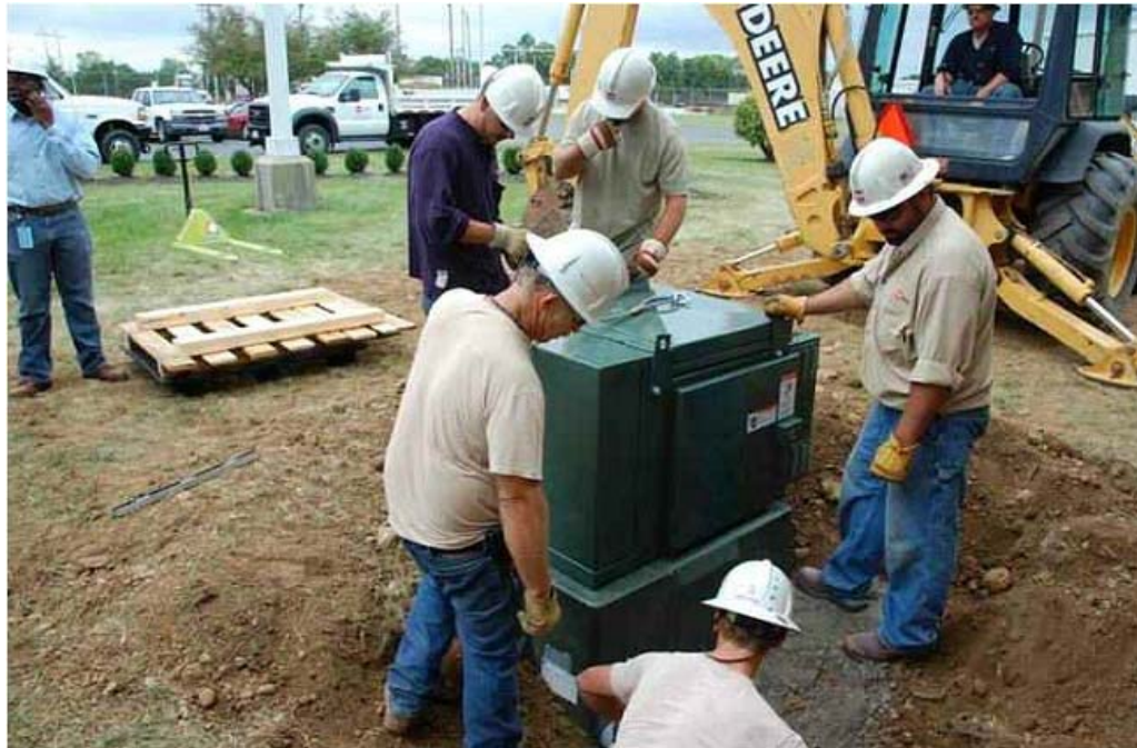
Figure H-4. Installing Above Ground 25 kW PCS Portion of CES
