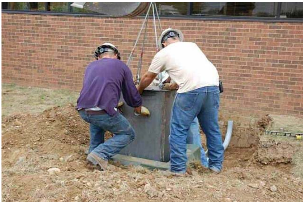
Figure H-3. Lowering 25 kWh Battery Container into Subterranean Vault
