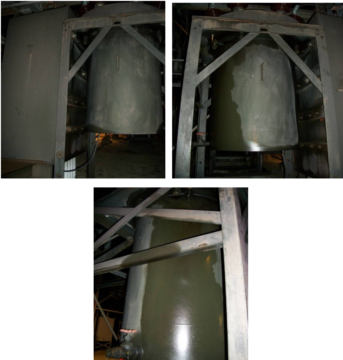
Figure 21: Circuit Breaker at Bathurst TS 85M4 (February 2, 2012)
