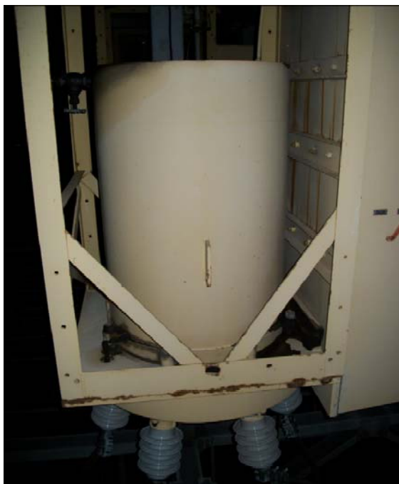
Figure 17: Circuit Breaker at Finch TS 55M24 (February 2, 2012)
