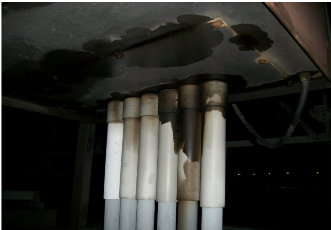
Figure 22: Circuit Breaker at Bathurst TS 85M2 (February 2, 2012)
