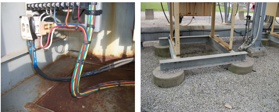
Figure 4: Circuit Breaker at Finch TS 55M28 (September 26, 2011)
