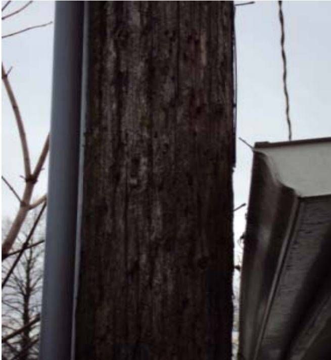
1 Figure 12a: Example of a rear lot pole close to an eavestrough (photo taken in 2012)
