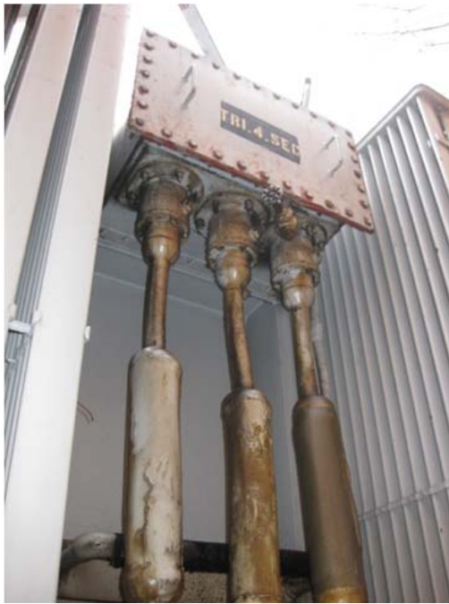
1 Figure 11: Transformer TR4 shows significant signs of oil leakage (note the oil saturated mats) 2 (January 16, 2012)
