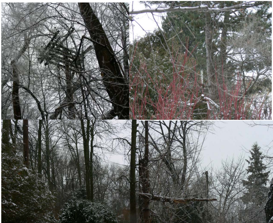
1 Figure 11: Vegetation encroaching on THESL assets in the Forest Hill, Banbury-Larkfield- 2 Charnwood, Livingston Guildwood, and Leslie-Lawrence rear lot area (photos taken in 2012)
