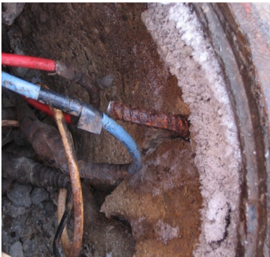
2 Figure 5 – Repaired Cable
