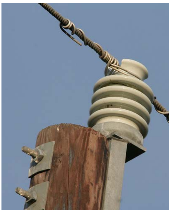
7 Figure 54: Typical Porcelain Insulator
