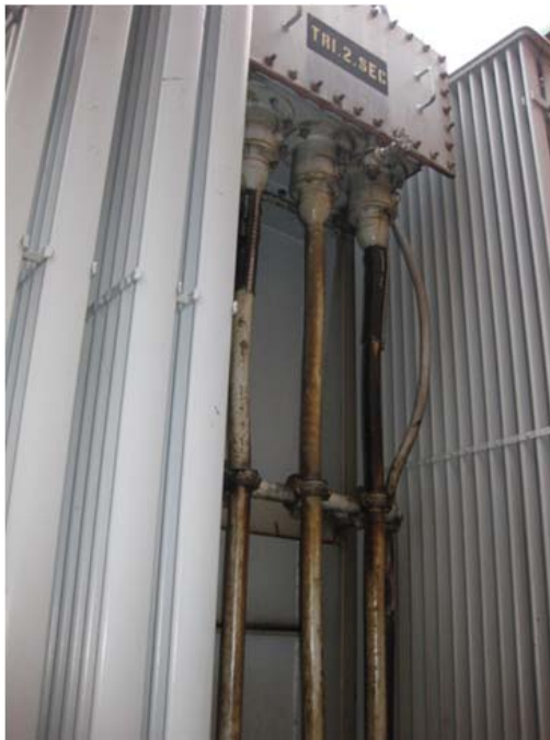
1 Figure 9: Transformer TR2 with more significant oil leakage (January 16, 2012)
