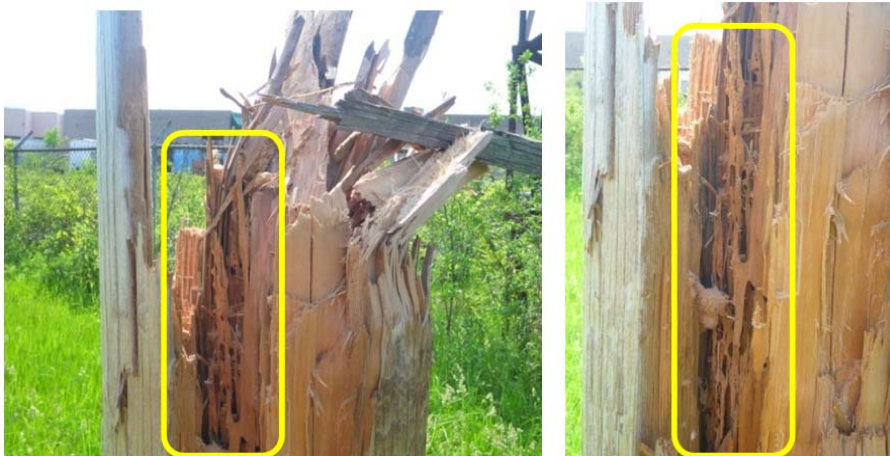
2 Figure 10: Evidence of Infestation
