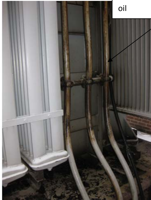
1 Figure 9: Transformer TR2 with more significant oil leakage (January 16, 2012)
