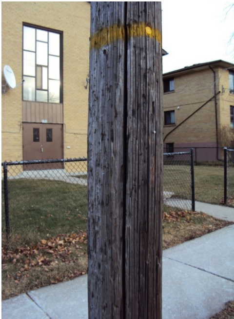
1 Figure 5: Pole cracks and holes
