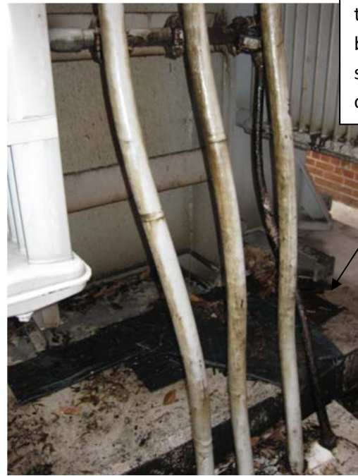
1 Figure 11: Transformer TR4 shows significant signs of oil leakage (note the oil saturated mats) 2 (January 16, 2012)
