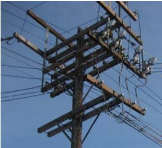
13 Figure 1: Typical Box Construction Installation (January 16, 2012)
