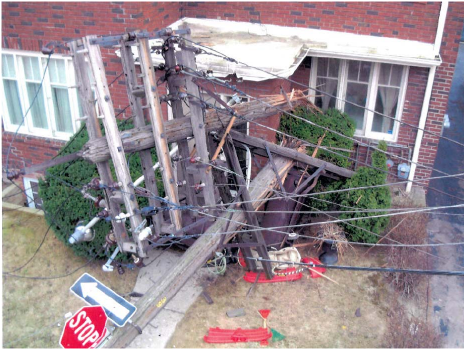
1 Figure 13: Pole Down on Acacia Road
