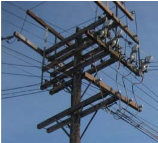
15 Typical Box Construction Installation (January 16, 2012)
