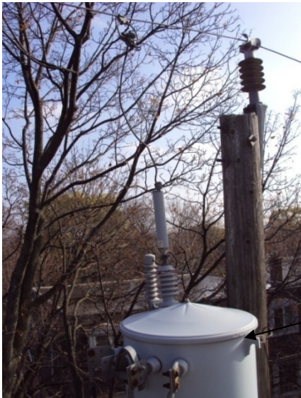
1 Figure 19: CSP Transformer
