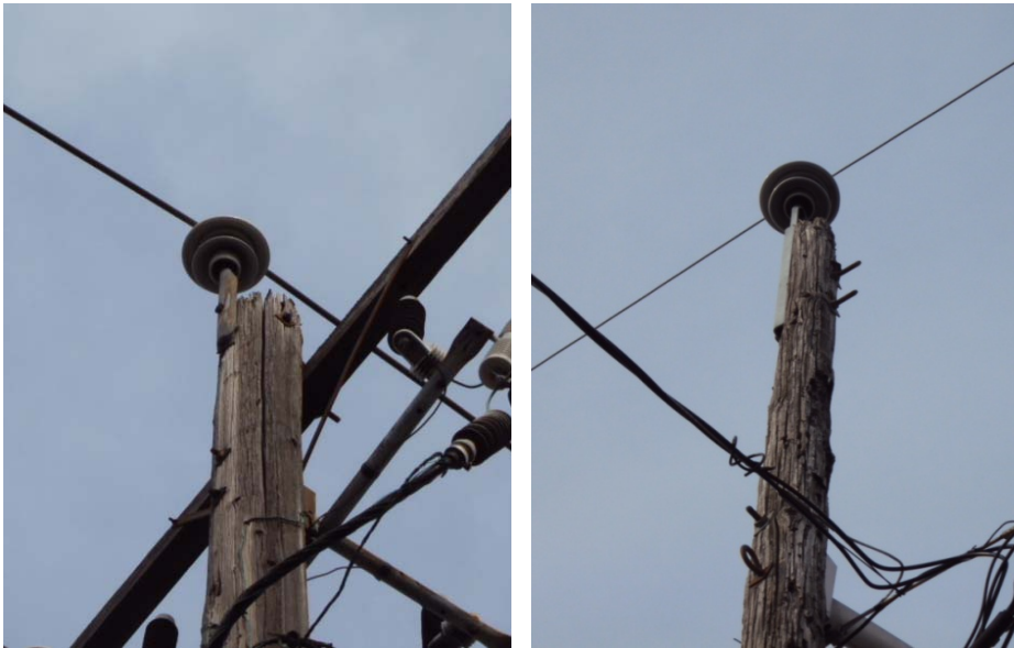
1 Figure 3: Pole-Top Feathering
