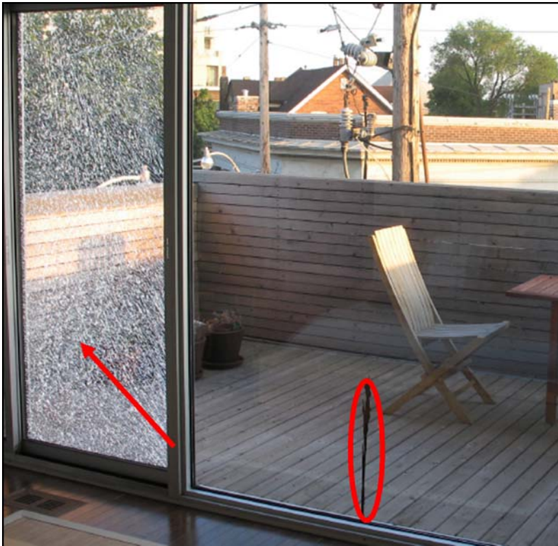
1 Figure 56: Failure Effects of the Porcelain Pothead Terminators 2
