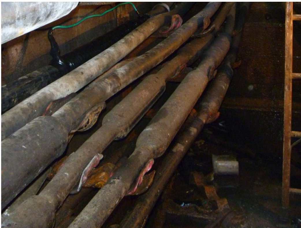
3 Figure 9: After — Cable Chamber showing properly supported cables and splices in a cable 4 rack within the cable chamber (January 18, 2012)
