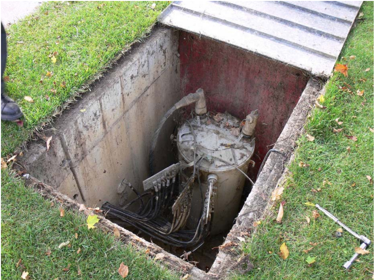
1 Figure 10 – Typical Submersible Transformer Vault
