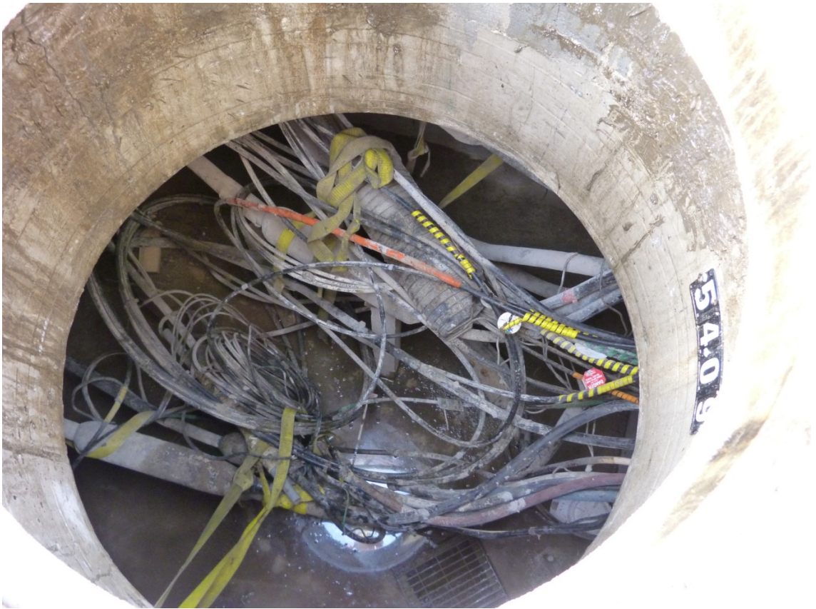
1 Figure 3: Chamber Requiring Piecing Out at Yonge and Merton (January 16, 2012)
