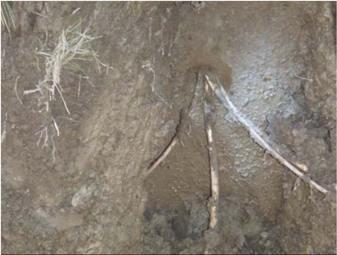
1 Figure B2: Typical environment of direct buried cables (taken on August 5, 2011)
