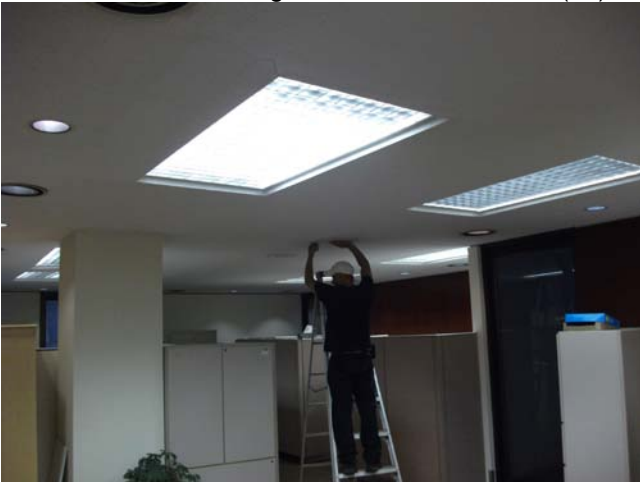
Photograph 15: [Rm. 16] View of newly-installed 1'x1' hatch (#2).
