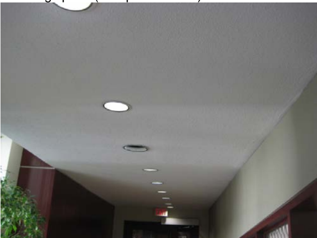
Photograph 5: [Rm. 6] White texture coat application (Sample set TH-4) applied over drywall ceiling.
