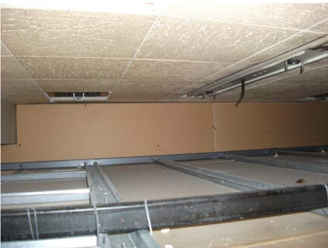
Photograph 17: [Rm. 16] View of ACT-2 on deck inside newly-installed hatch (#2).
