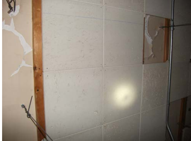
Photograph 8: [Rm. 8] 1'x1' acoustic ceiling tiles (ACT-2) in the ceiling space.
