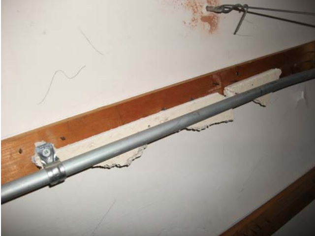
Photograph 7: [Rm. 1] 1'x1' acoustic ceiling tile (ACT-2) debris in the ceiling space (Sample set TH-3).
