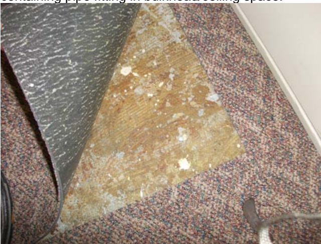
Photograph 11: [Rm. 10] View of concrete and underpad adhesive underneath carpet.
