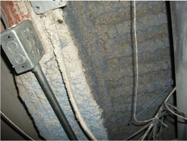
Photograph 3: [Rm.5/7] Sprayed fibrous fireproofing in ceiling space (Sample set TH-5).
