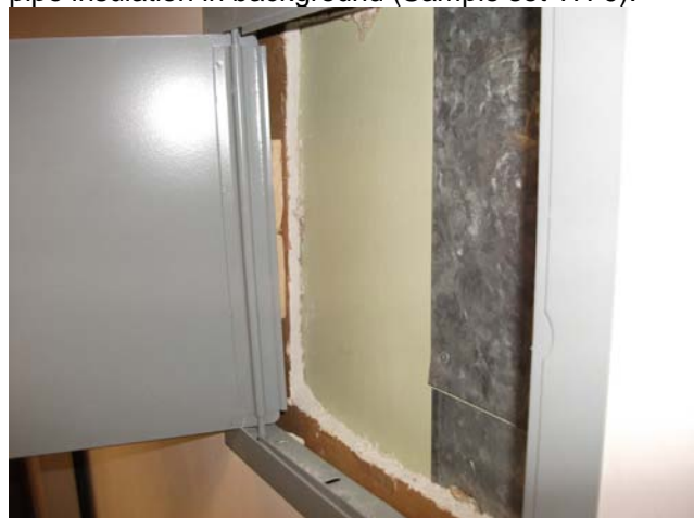
Photograph 18: [Rm. 1] View of double-layered drywall inside newly-installed hatch (#4).
