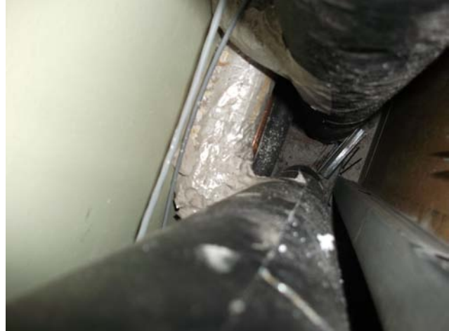
Photograph 14: [Rm. 6] View inside newly-installed hatch (#1) (no visible asbestos-containing materials).
