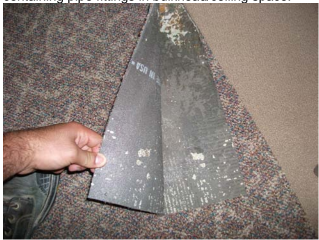
Photograph 12: [Rm. 9] View of concrete and underpad adhesive underneath carpet.
