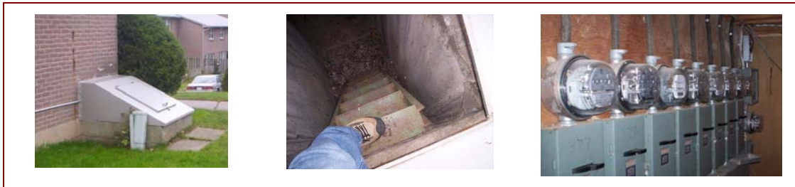
Figure 5-7, Typical Arrangement of Subsurface Electrical Room
