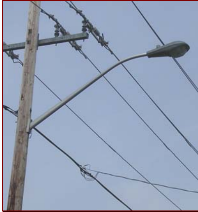
Figure 6-4, Cobra-Head Luminaire for Main Streets
