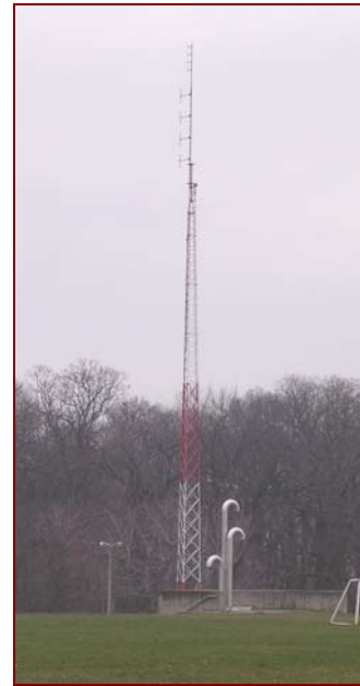
Figure 6-10, Springbank Reservoir Radio Tower
