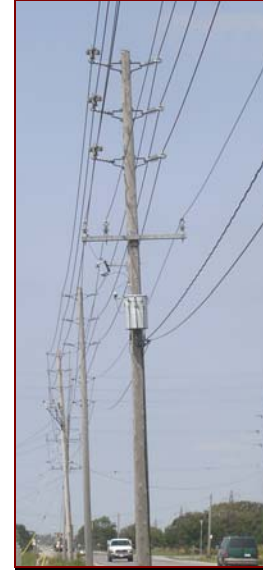
Figure 6-13, Typical Three-Circuit Aerial Construction
