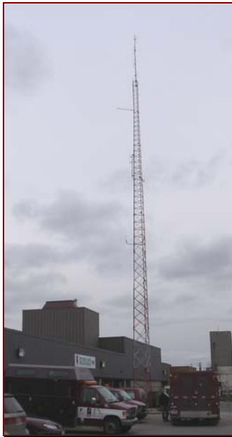
Figure 6-8, Head Office Radio Tower
